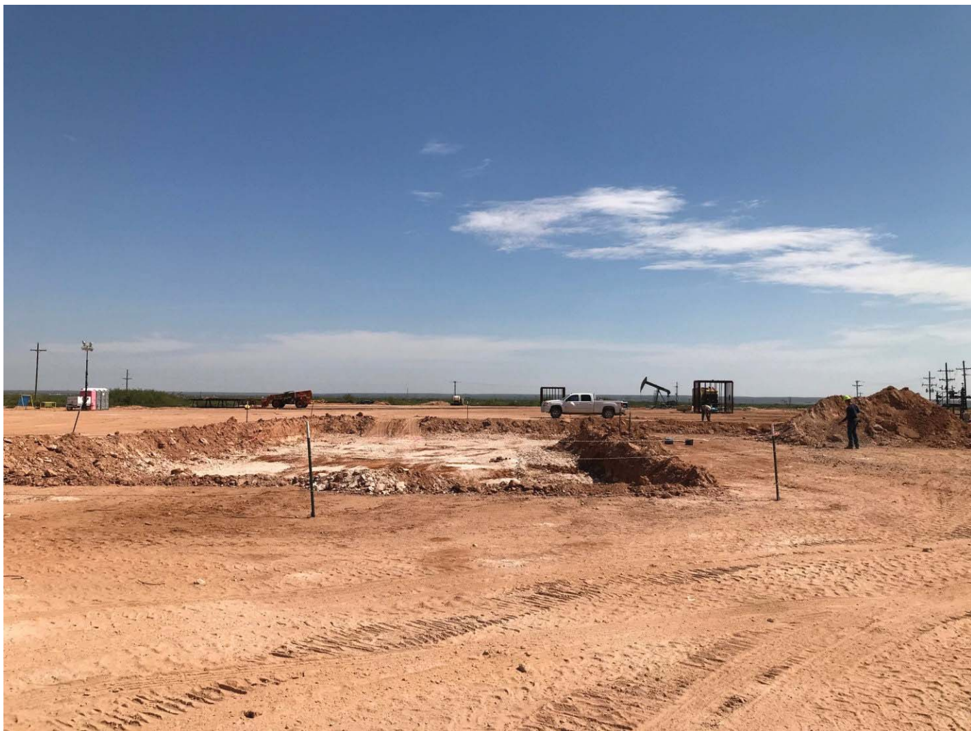
Southern view of final excavation extent during confirmation soil sampling activities.
