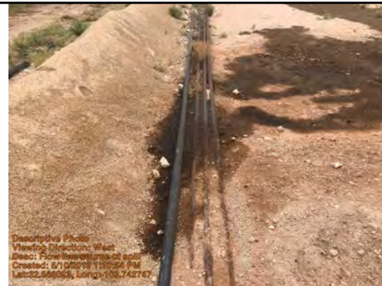
Flow line source of spill
