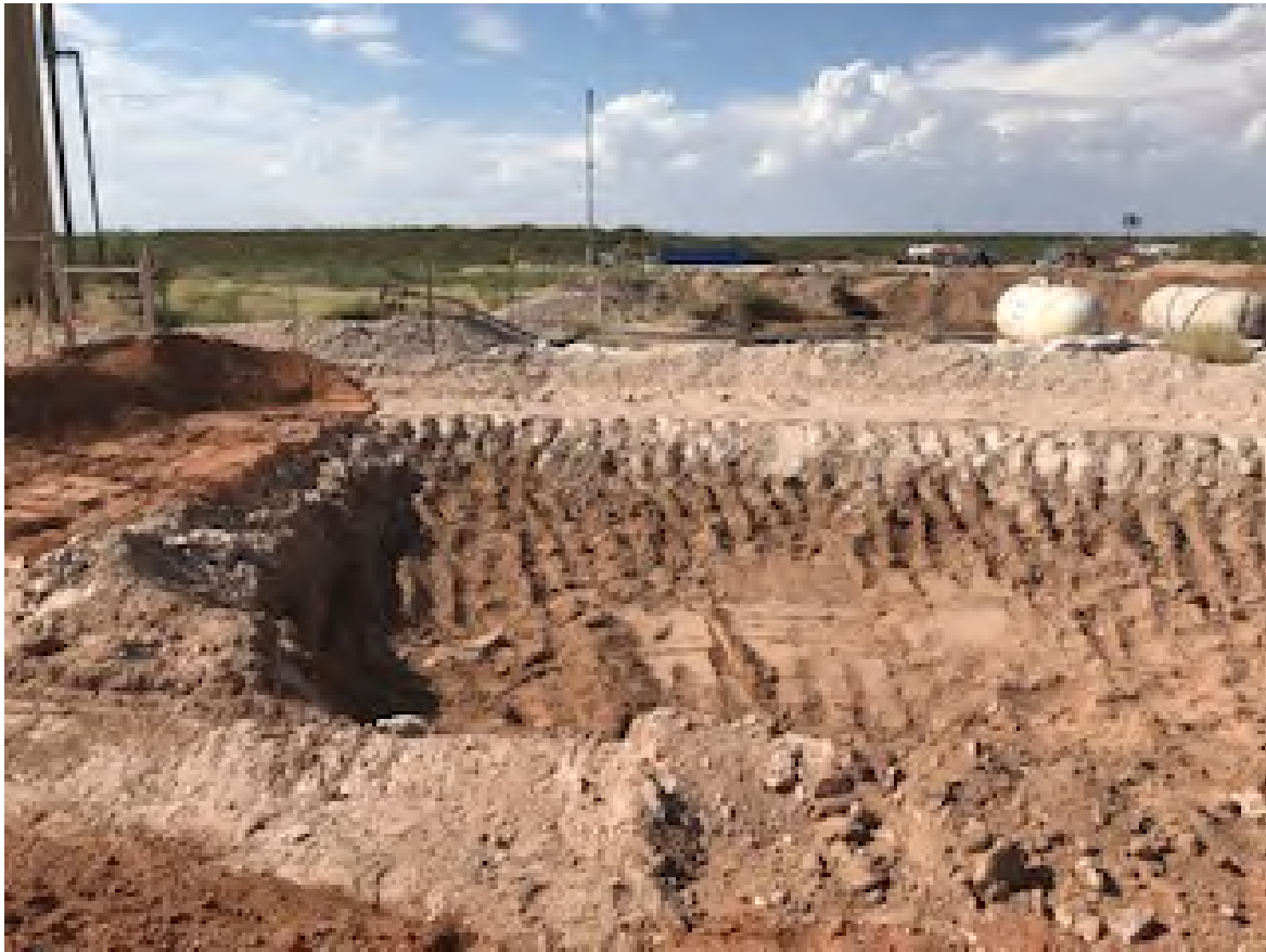
North facing view of the excavation on the well pad.
