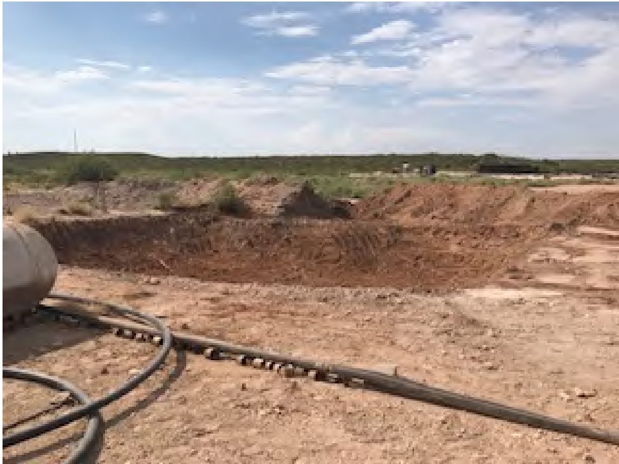
North facing view of the western excavation.
