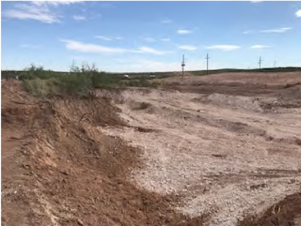
North facing view of the excavation northeast of the well pad.
