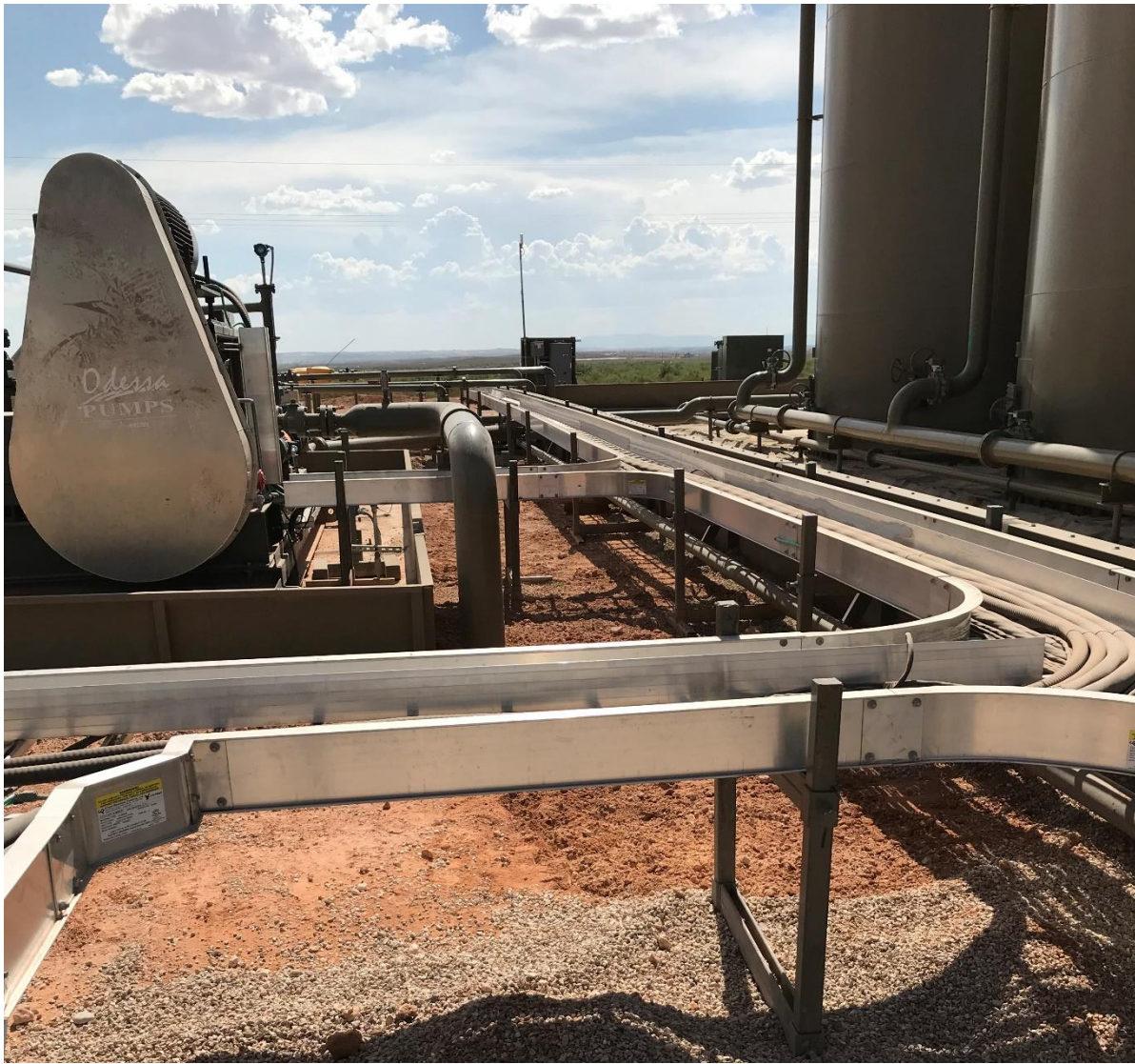
Western view of July excavation extent.
