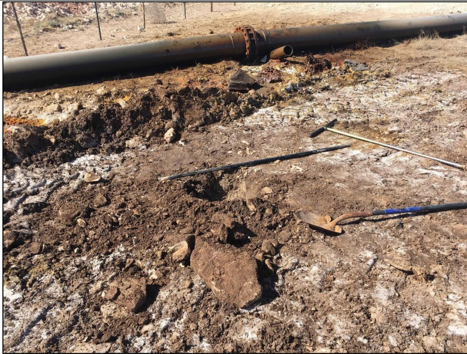
PHOTO 3: View of HA-1, Facing West. 3/01/2019
