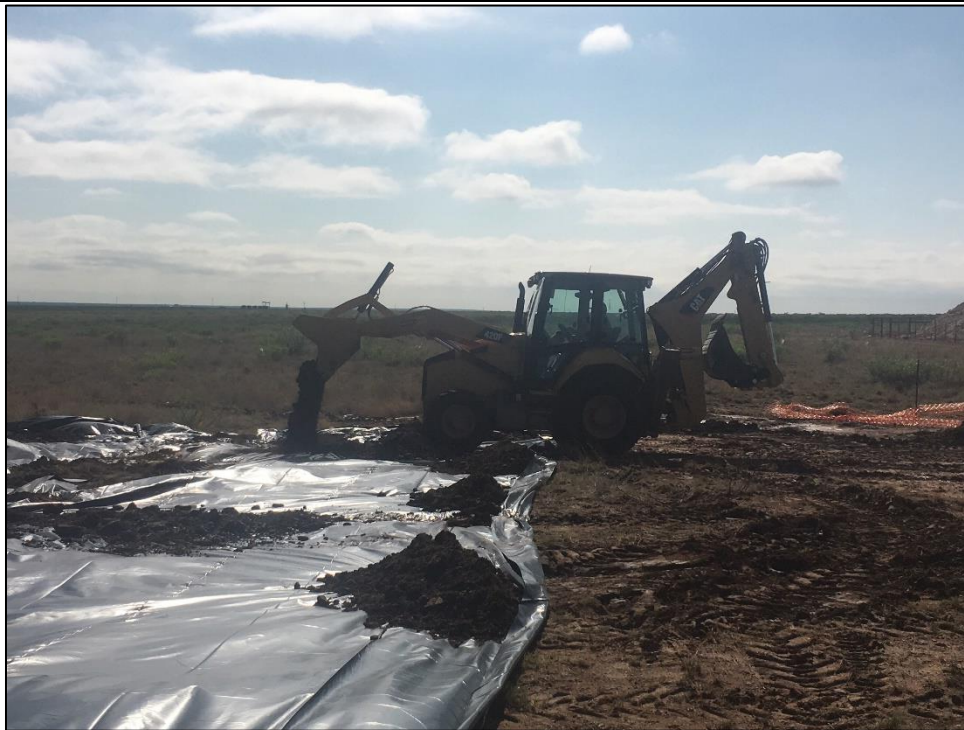
PHOTO 15: View of Remediation Activity, Facing East. 6/04/2019
