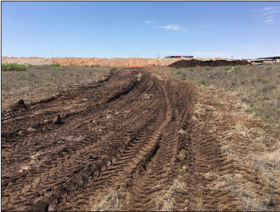
PHOTO 29: View of Remediation Activity, Facing South. 6/05/2019
