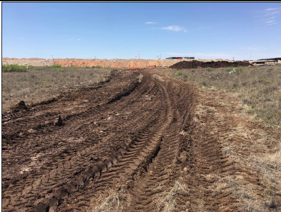
PHOTO 16: View of Remediation Activity, Facing South. 6/05/2019
