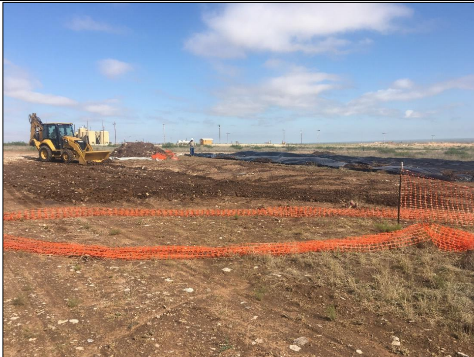
PHOTO 14: View of Remediation Activity, Facing West. 6/04/2019
