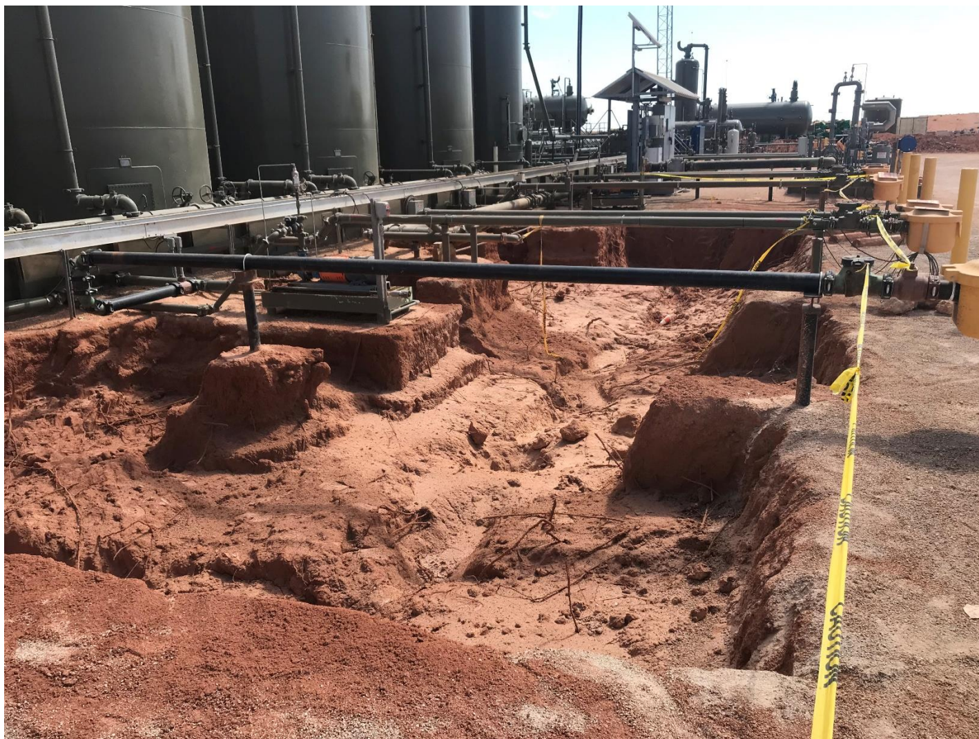
Eastern view of final excavation extent during confirmation soil sampling activities.
