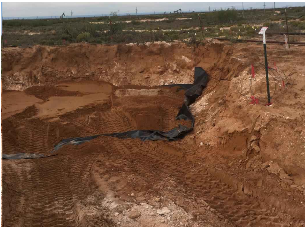
View East – Area being backfilled with liner installed
