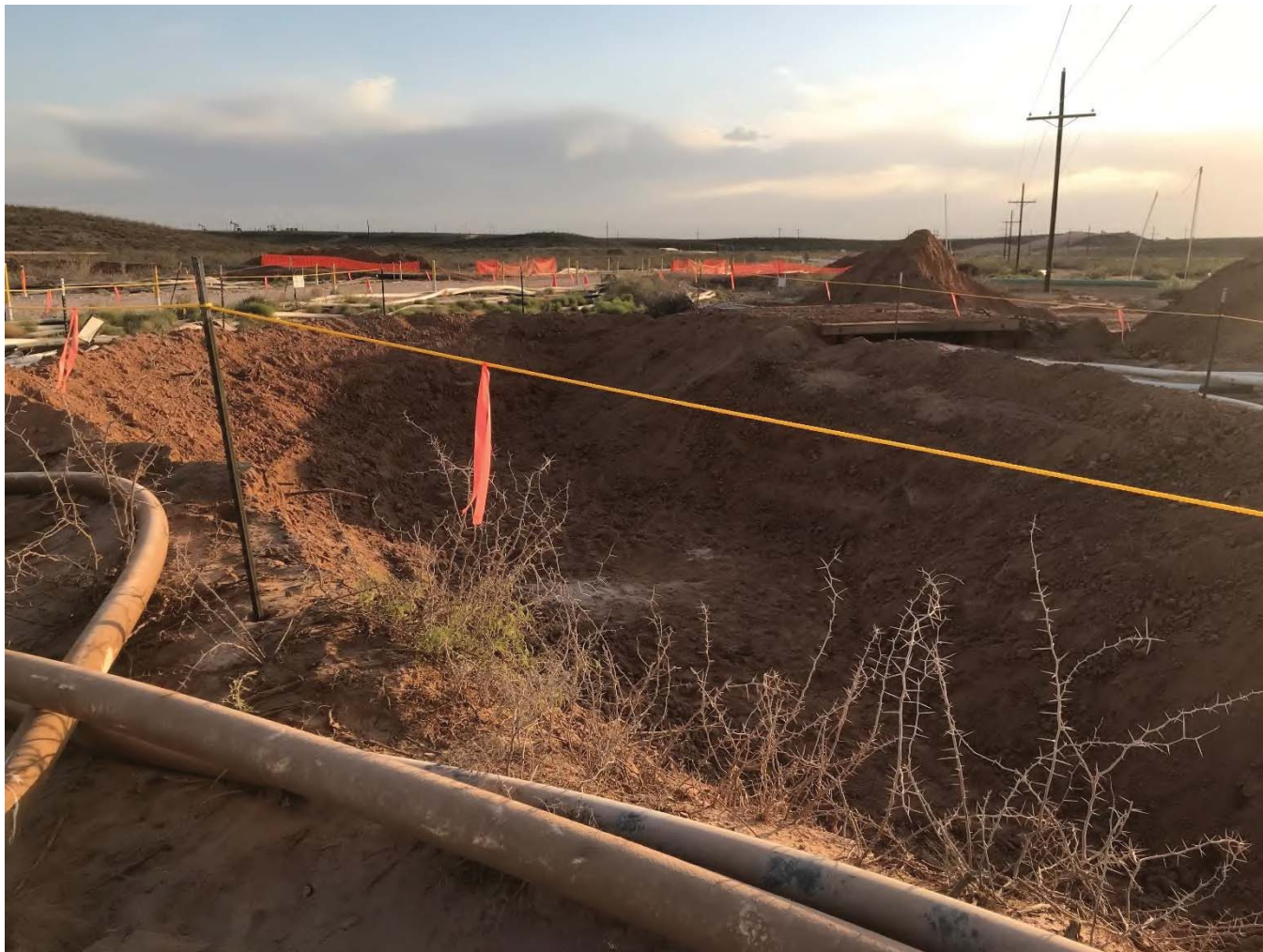
Northern view of final excavation extent.
