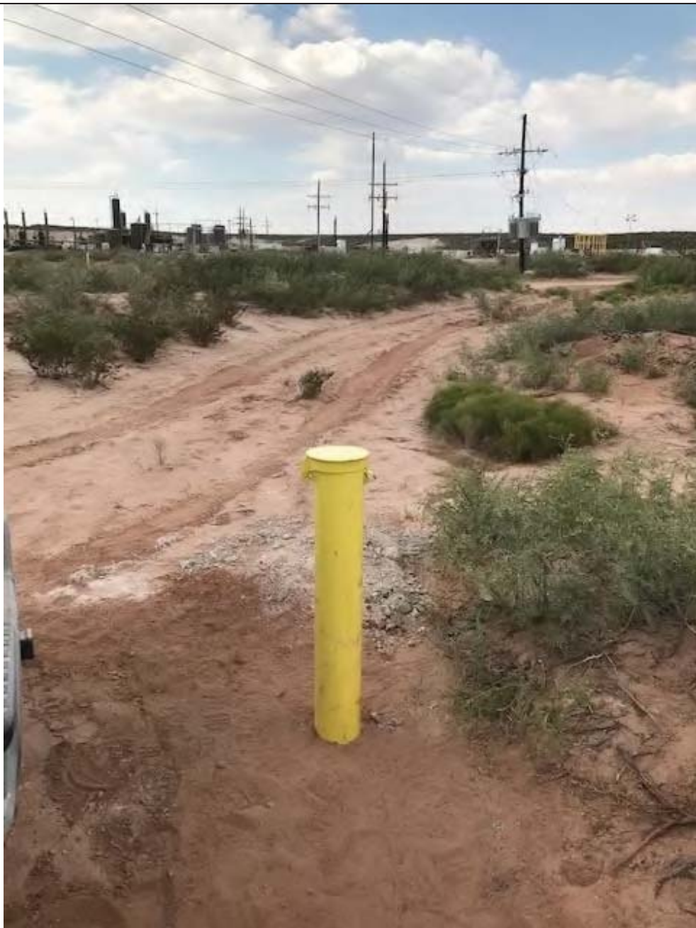
Northern view of groundwater monitoring well MW05 after installation and development.
