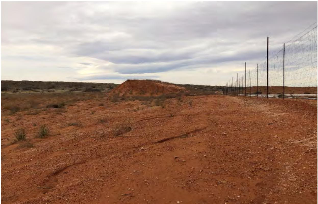
*Figure 2 - Topsoil stockpile for existing Dagger Pond in the NW corner of Dagger 2 site.*
