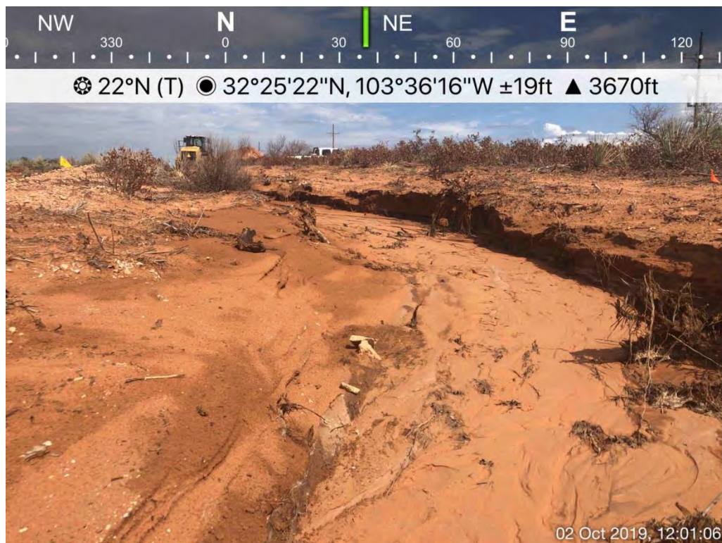
Water Eroded Channel Viewing Northeast, October 2, 2019
