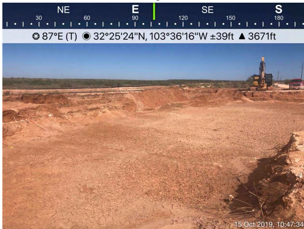
DP-1 and DP-2 Excavations Viewing Northwest, October 15, 2019
