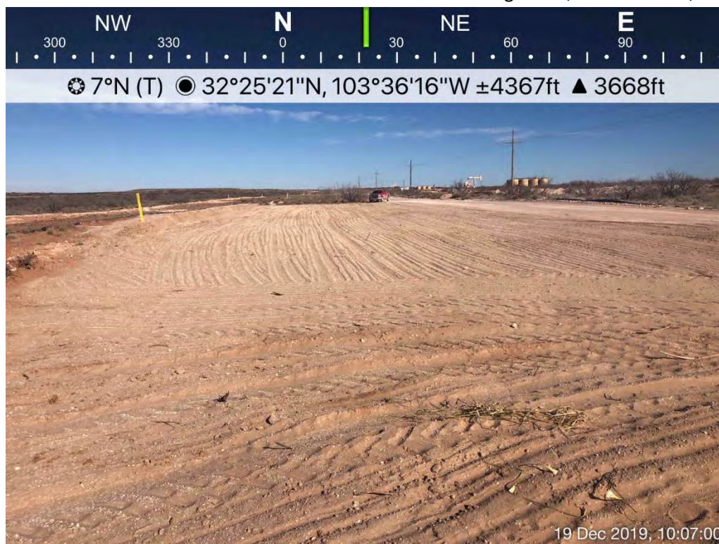
Backfilled and Seeded DP-1, DP-2, and DP-3 Excavation Area Viewing North, December 19, 2019
