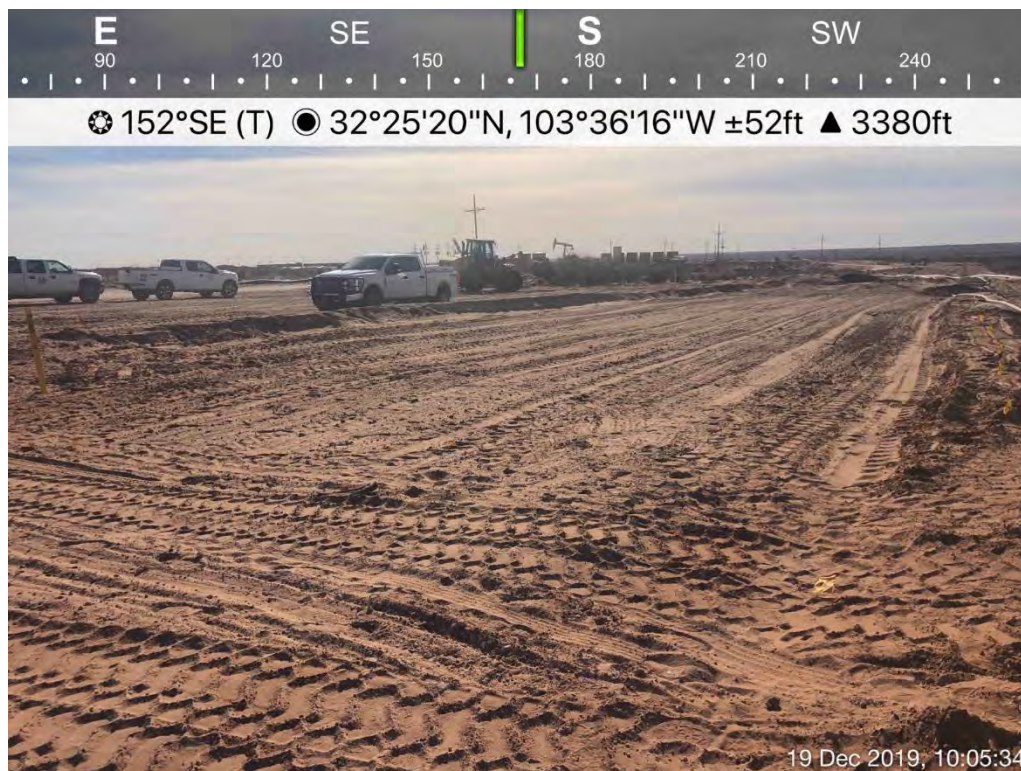
Backfilled and Seeded HA-5 and HA-6 Excavation Area Viewing South, December 19, 2019
