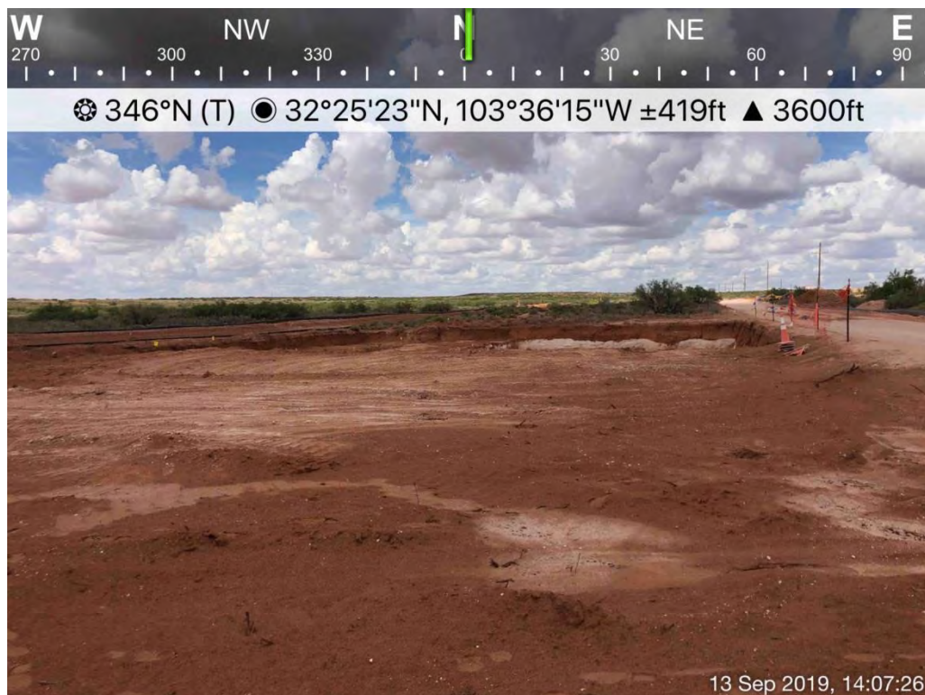
DP-1, DP-2, and DP-3 Excavations Viewing North, September 13, 2019
