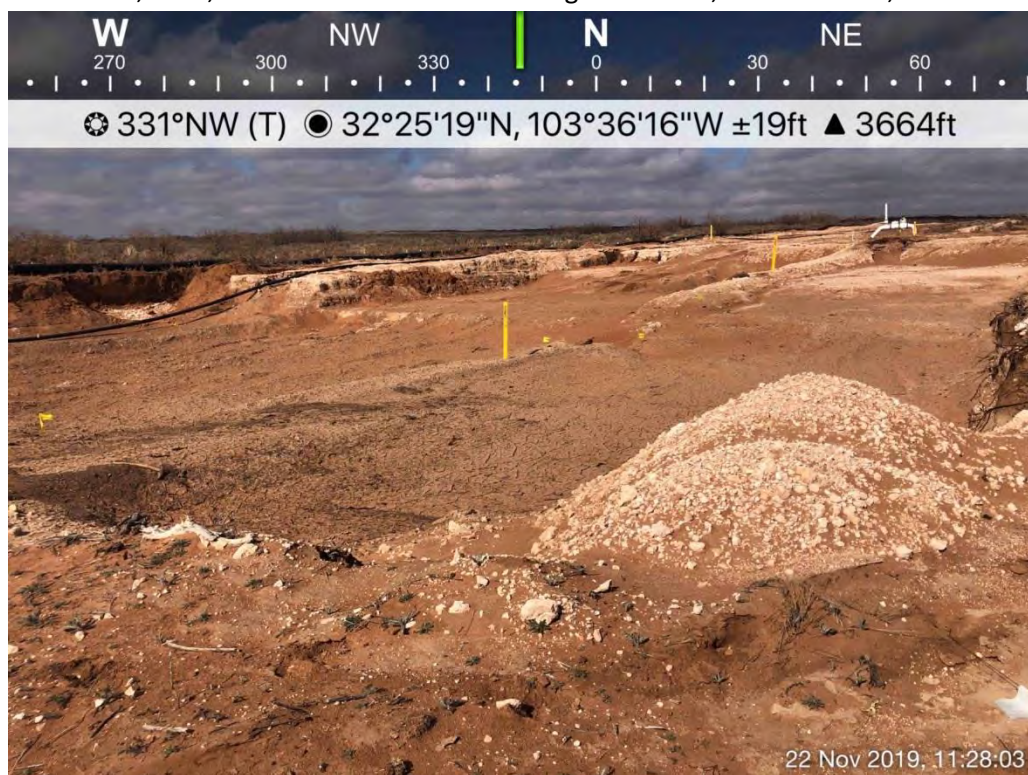
HA-5 and HA-6 Excavations Viewing Northwest, November 22, 2019
