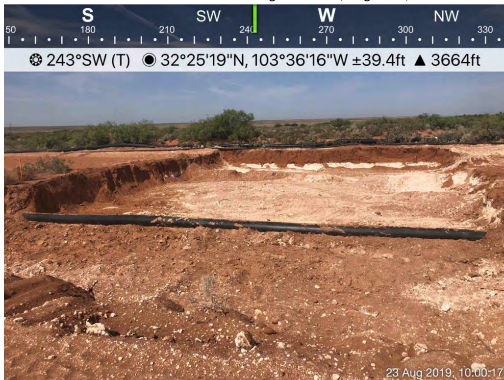
HA-5 Excavation Viewing West, August 23, 2019
