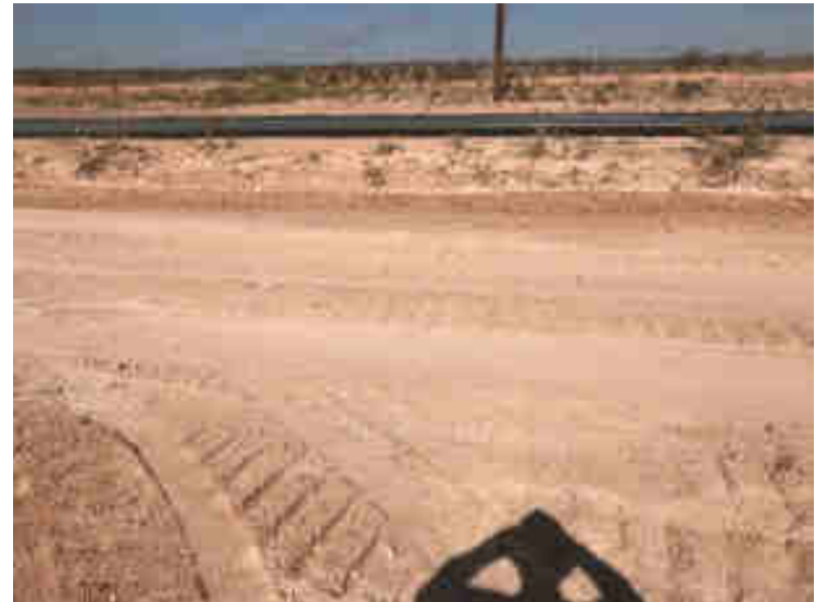
Photograph 8: View north of lease road after scraping road.
