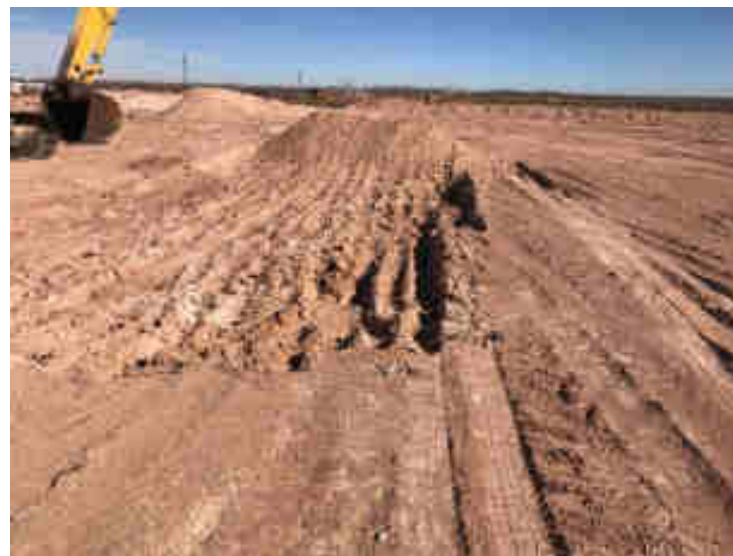
Photograph 4: View of the excavation on the pad facing east.
