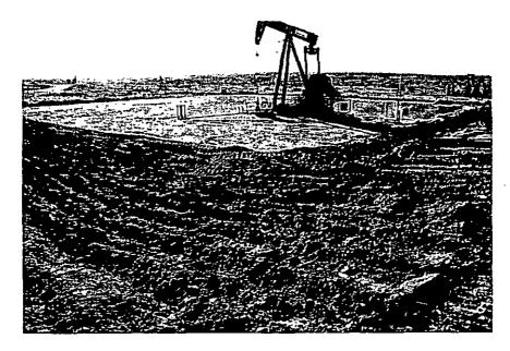
Corners rounded off to gain more in reclamation since these areas are not used for daily operations. IR followed plan in AAPD with IR added to the south side taking to a 3:1 slope. Pad is bermed.
