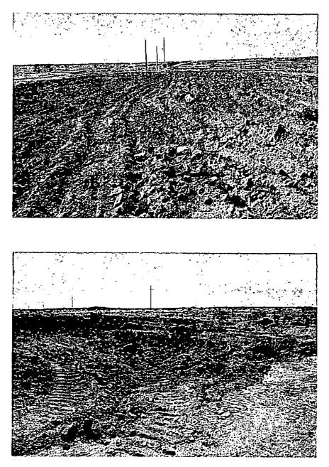
Corners rounded off to gain more in reclamation since these areas are not used for daily operations. Extra reclamation was completed on the east to make up for loss of some acreage to the north due to new pipeline installation ROW. It didn't make sense to reclaim this area. Reclaimed area was moved to the south and east to close out some pasture. This was also the deepest area of cut that needed to be backfilled with material taken from the west.
