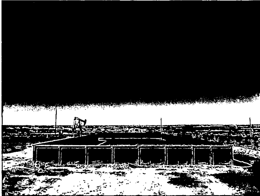
Firewall for SWD being constructed.
