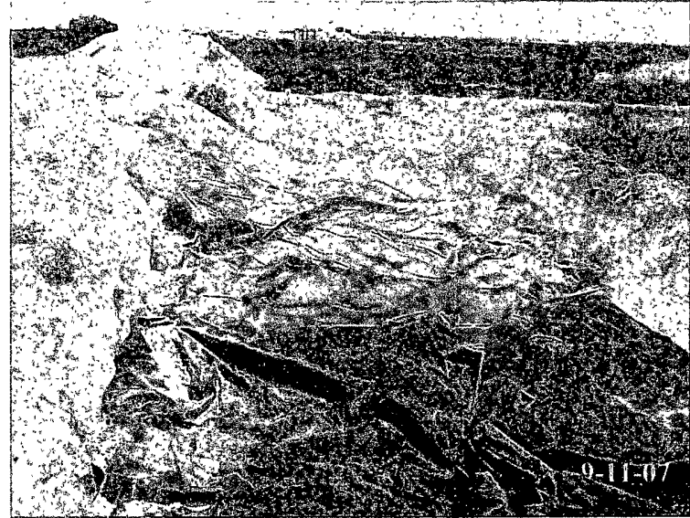
20 mil cap on bottom point that did not meet NMOCD standards.
