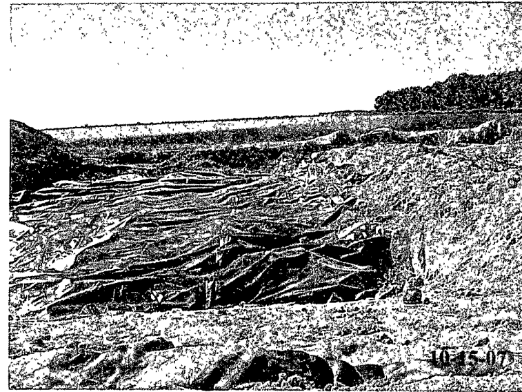
Burial pit capped with a 20 mil impervious liner.
