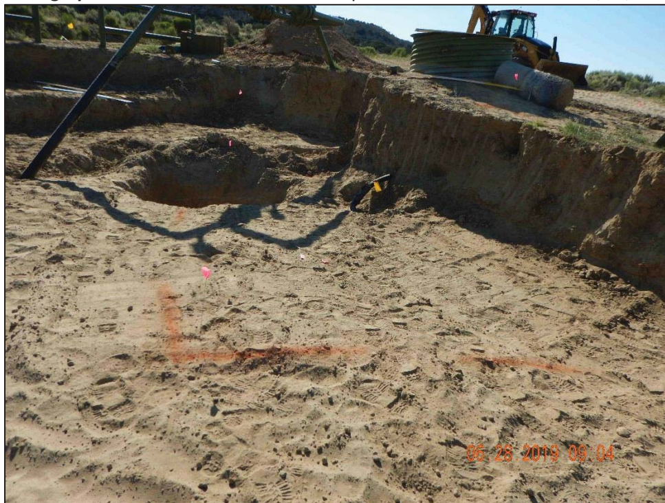
Photograph 15: Remediated Area and Sample Grid: SPF 34 and SW 13 - 6/28/19
