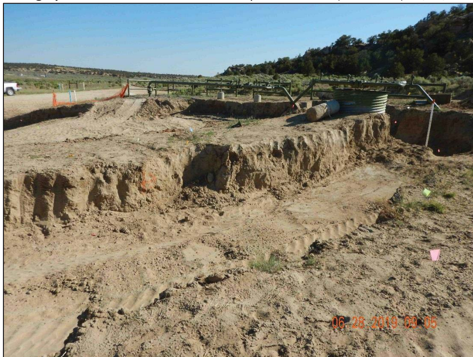
Photograph 17: Remediated Area and Sample Grid: SW 6 (SE Portion) - 6/28/19
