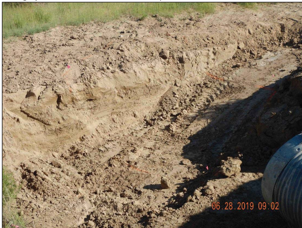
Photograph 13: Remediated Area and Sample Grid: SPF 2 - 6/28/19
