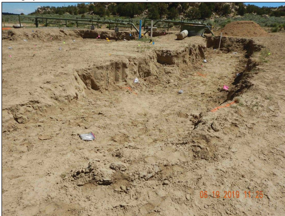
Photograph 8: Remediated Area and Sample Grid on Hillside SE of 208 Receiver – 6/19/19
