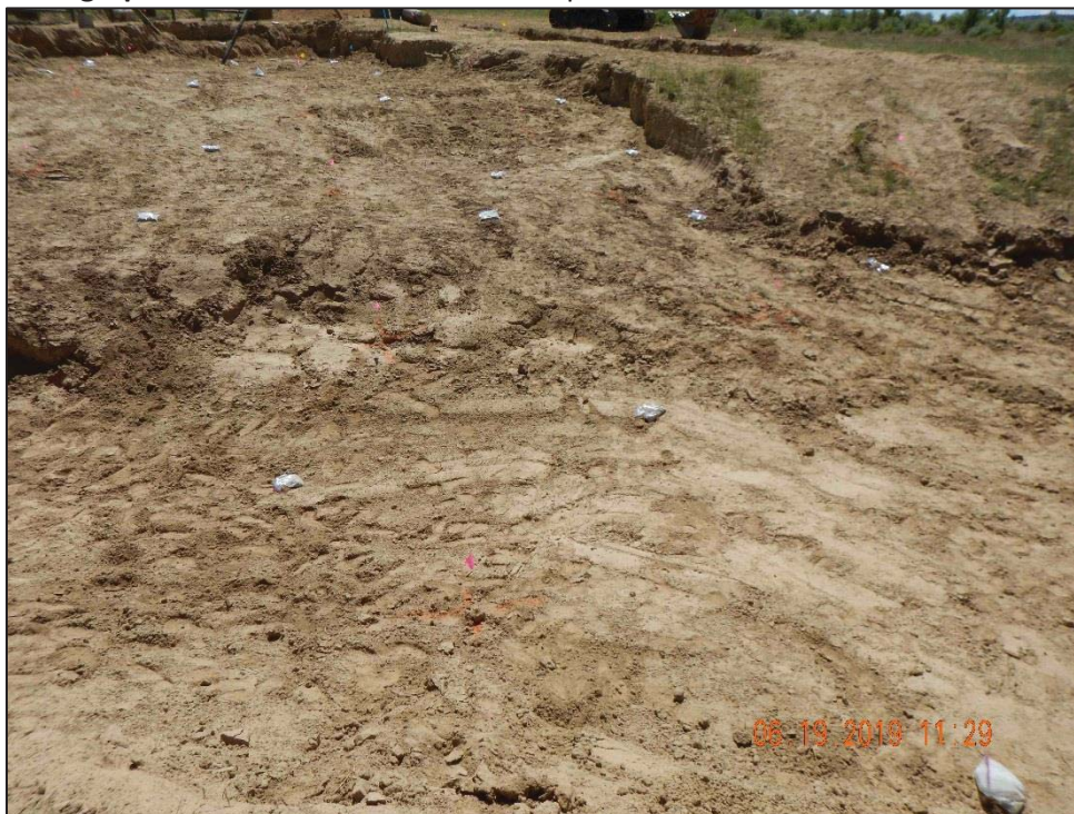
Photograph 10: Remediated Area and Sample Grid on Hillside SW of 208 Receiver – 6/19/19
