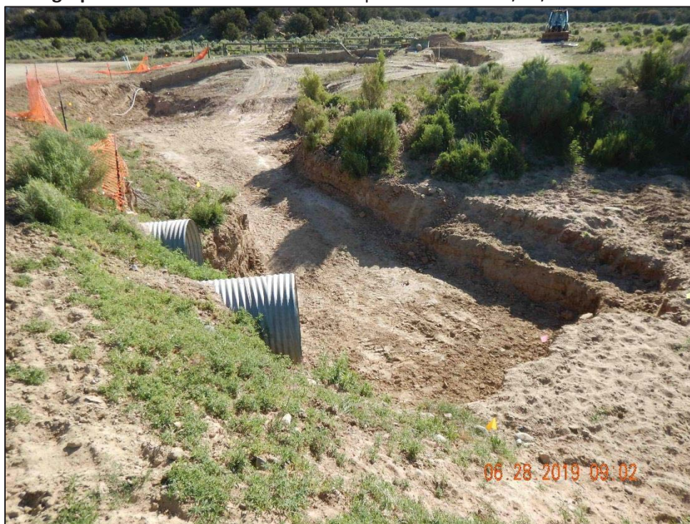
Photograph 18: Remediated Area and Sample Grid: SW 8 - 6/28/19
