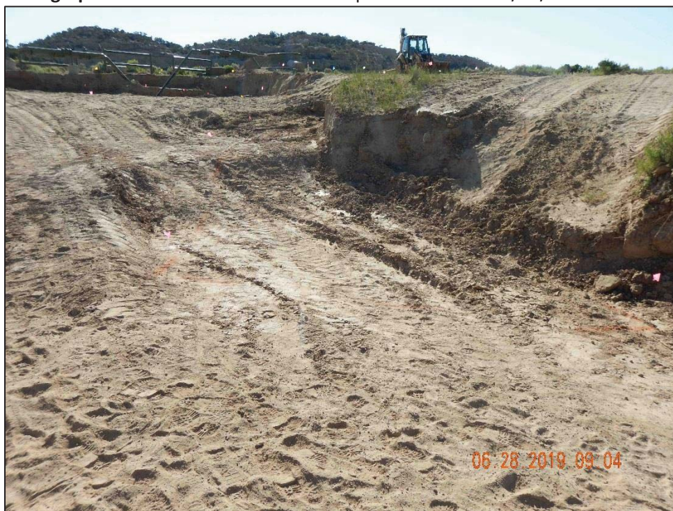
Photograph 14: Remediated Area and Sample Grid: SPF 21 - 6/28/19
