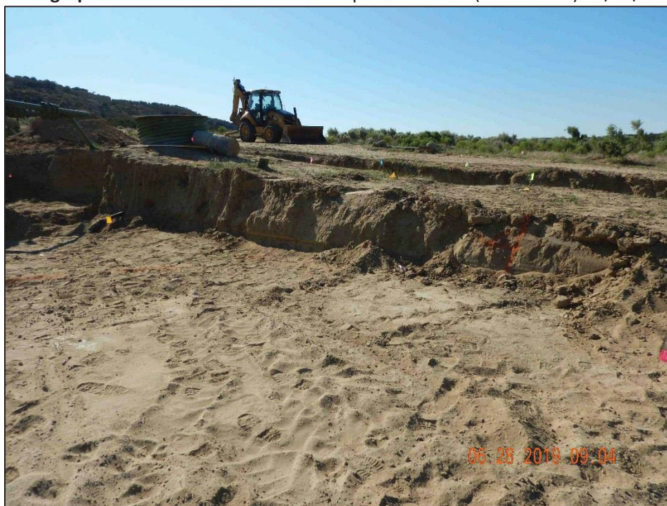
Photograph 16: Remediated Area and Sample Grid: SW 6 (SW Portion) - 6/28/19
