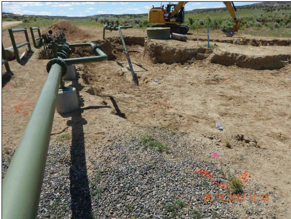
Photograph 7: Remediated Area and Sample Grid Adjacent to Point of Origin – 6/19/19
