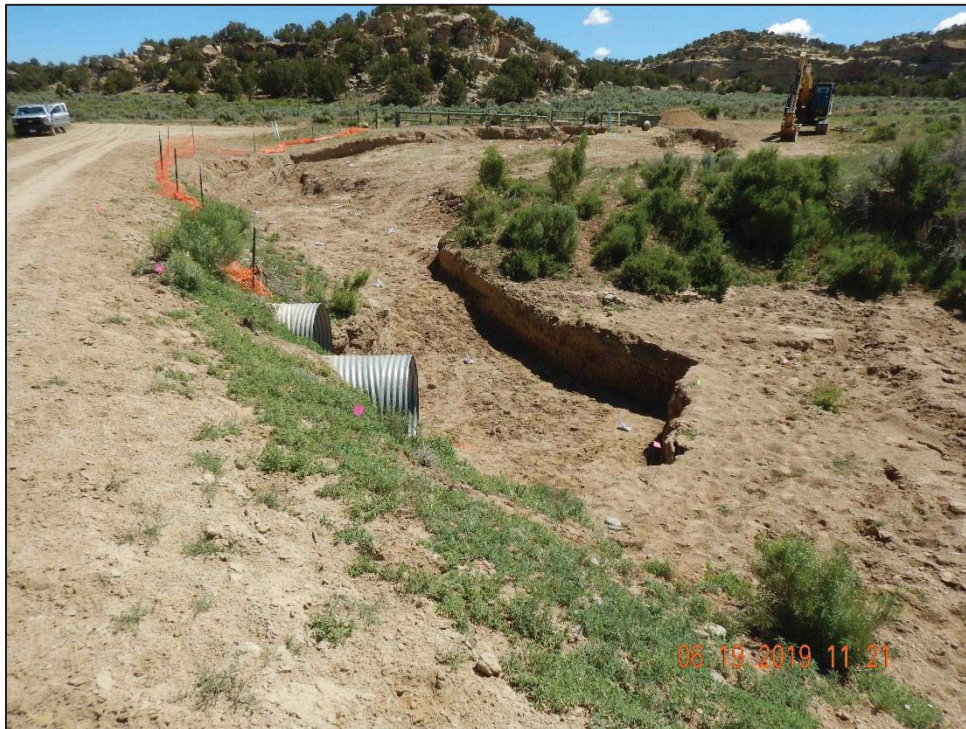
Photograph 11: Remediated Area and Sample Grid in Drainage; Up-Gradient – 6/19/19
