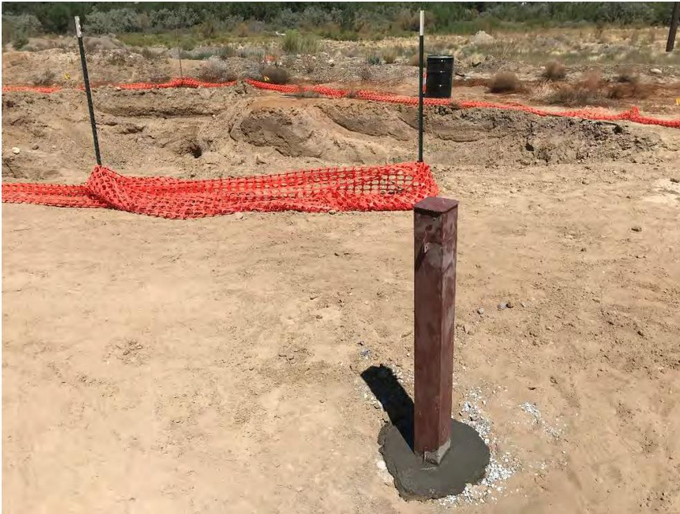
**Photograph 2:** MW05 completed well, 35 feet.
