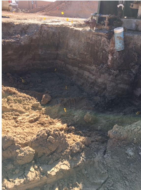
Photograph 1: Release location near well head, excavation 8 feet deep.
