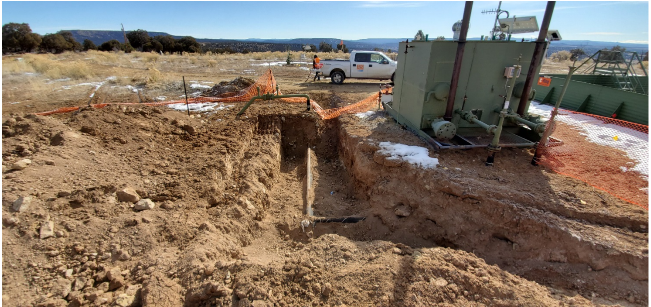
Photo 1: Excavation Area (21' x 11' x 5' to 6' deep).
