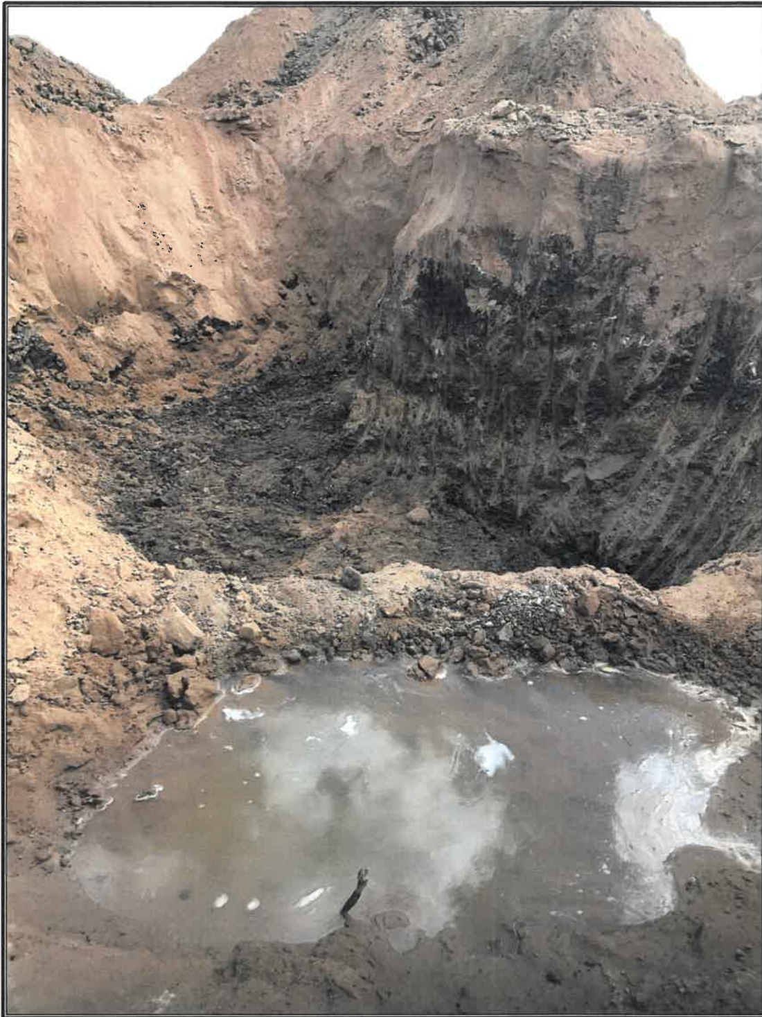
Photo 1: Site after Final Excavation Sampling
