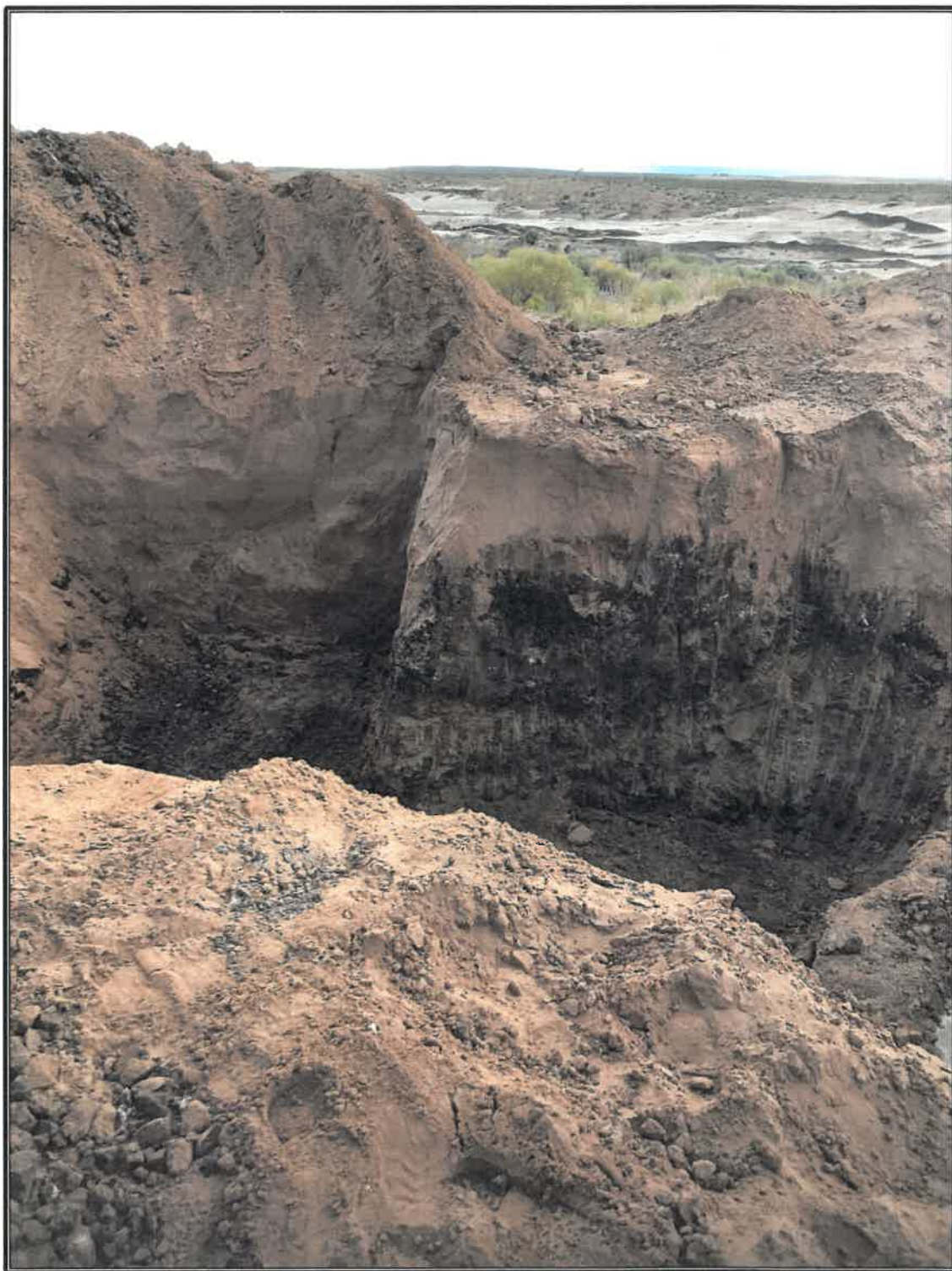
Photo 2: Site after Final Excavation Sampling (View 2)
