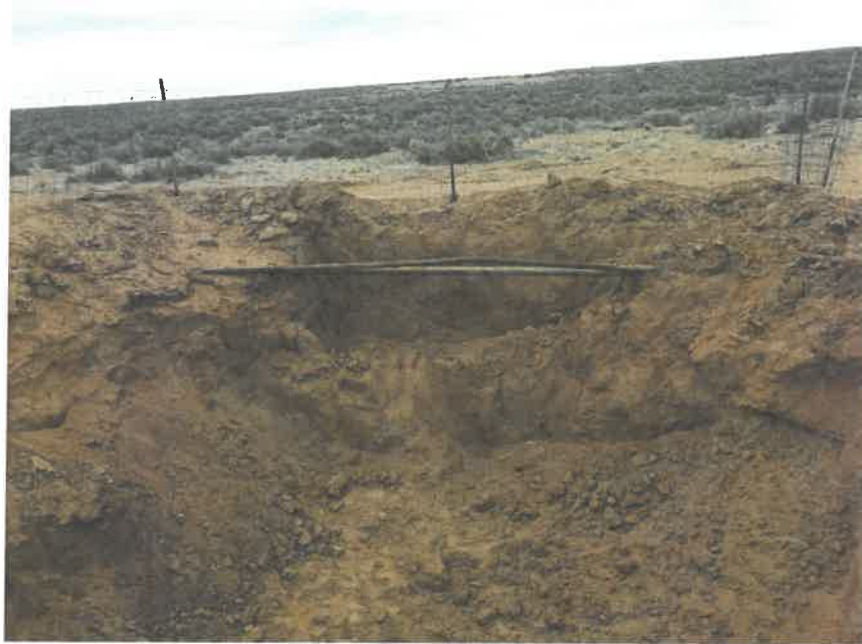
Photo 1: BGT excavation facing northeast. Photo taken December 21, 2018.
