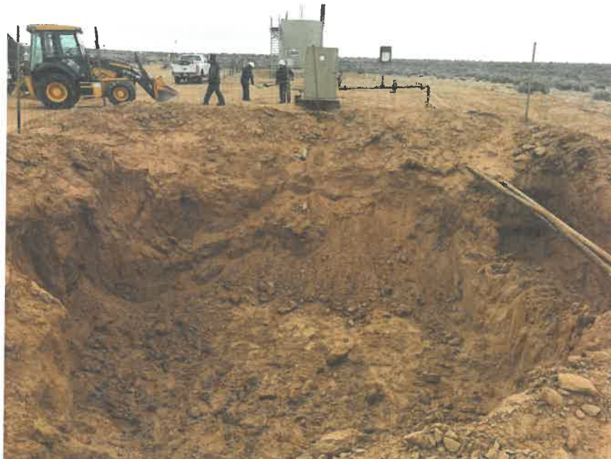
Photo 2: BGT excavation facing northwest towards the separator. Photo taken December 21, 2018.
