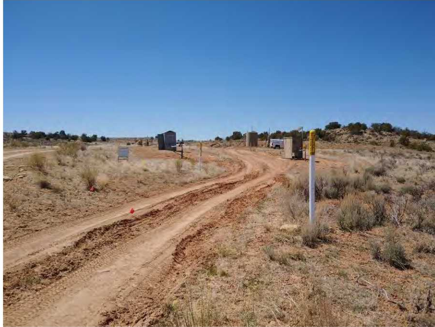
Figure 13. Measurement equipment to be removed and pipeline to be cut and capped in foreground.
