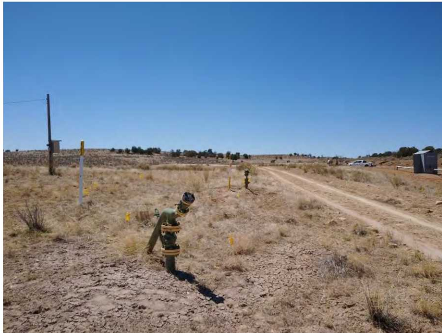
Figure 4. Enterprise doglegs to remain. Well-connect pipeline to dogleg in the background will be removed.
