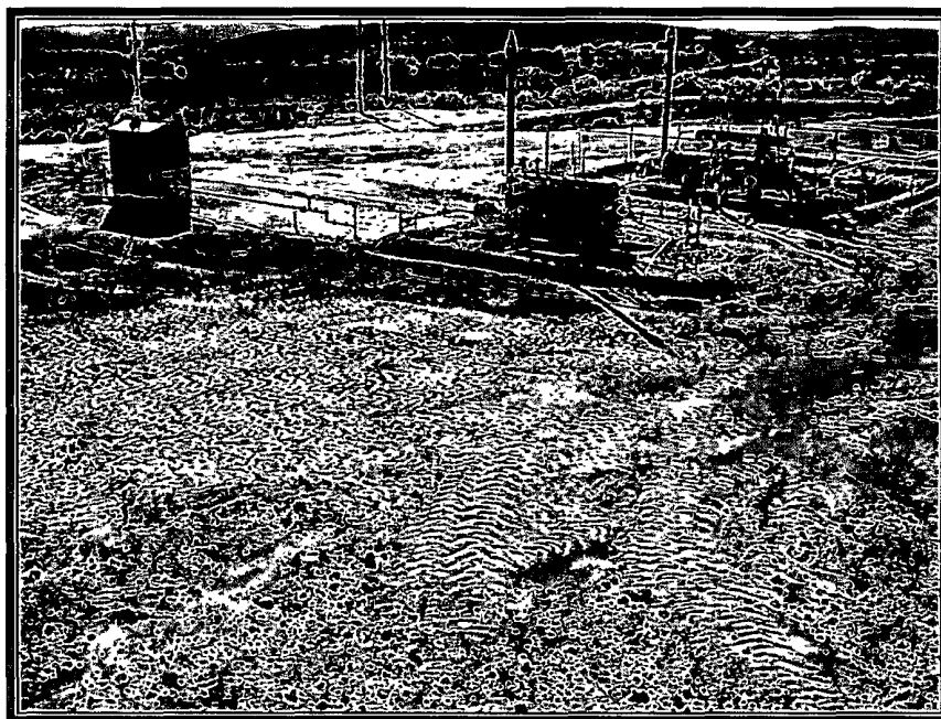
Photograph 4: Below Grade Tank Pit (Backfilled and Re-contoured)
