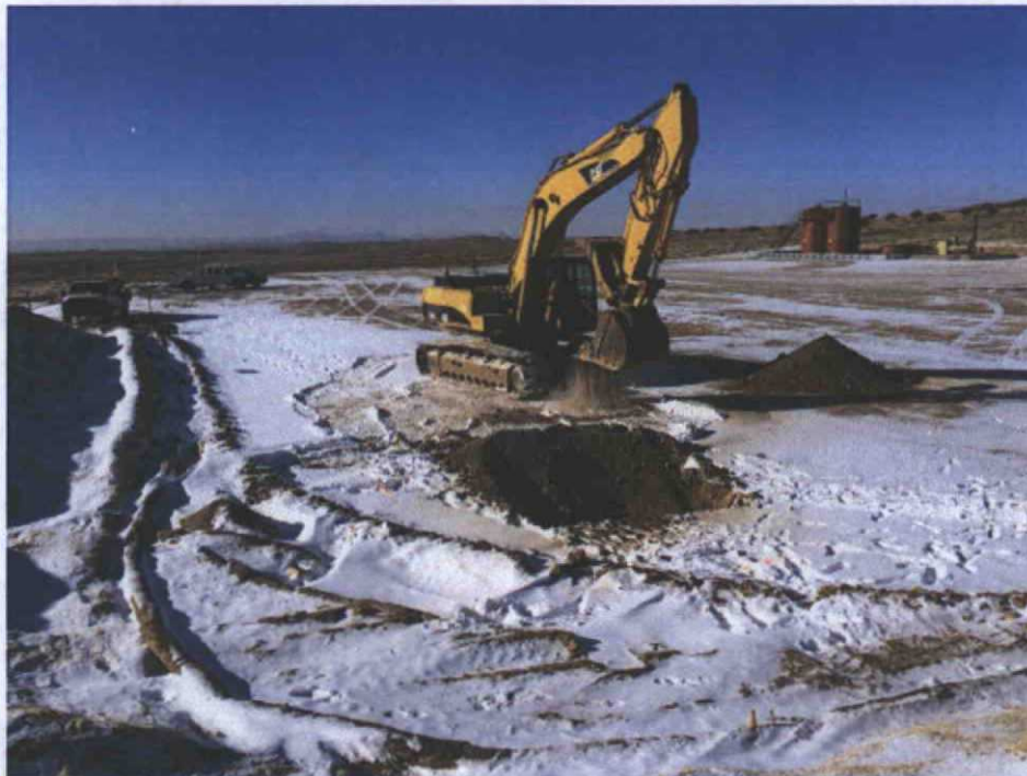
Figure 1: Excavating the cuttings trench.
