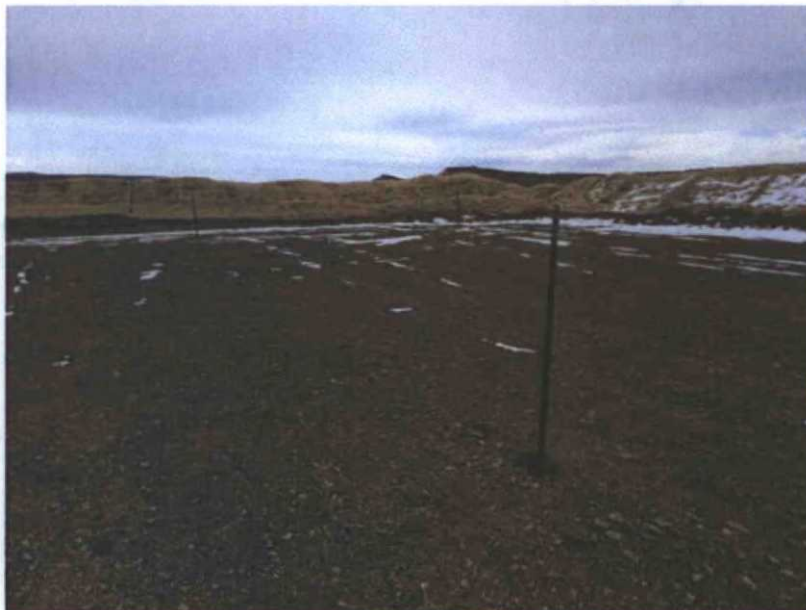
Figure 1: T-Posts placed at each corner of cuttings trench.
