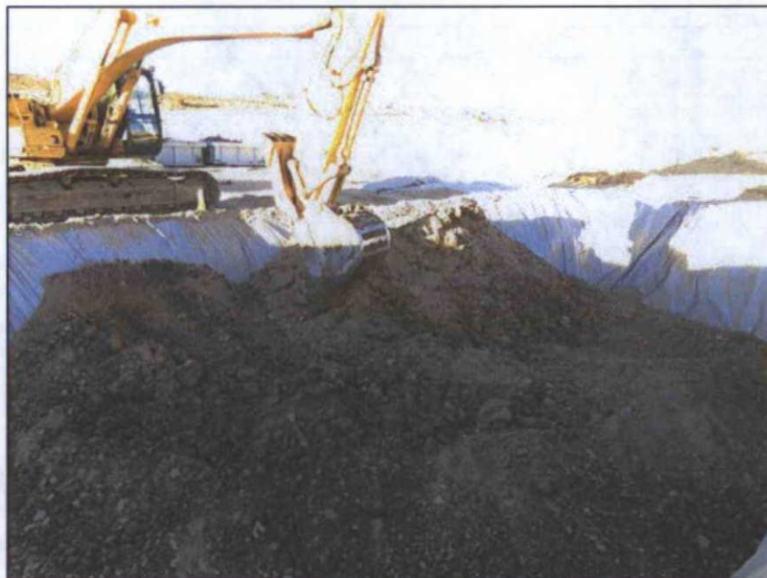
Figure 4: Spreading the mixed cuttings in the burial trench.
