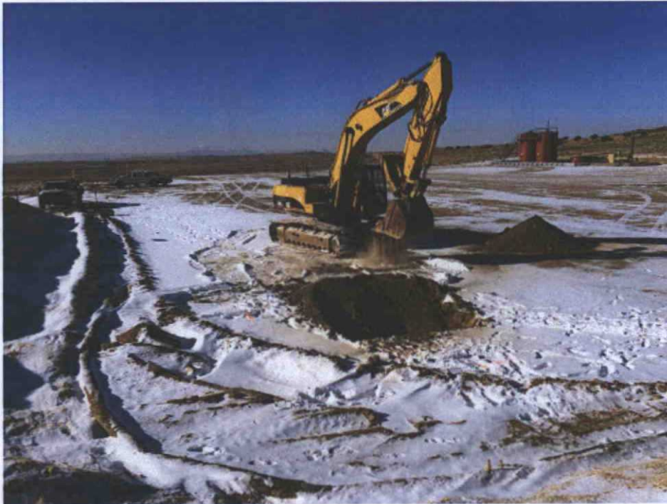
Figure 1: Excavating the cuttings trench.
