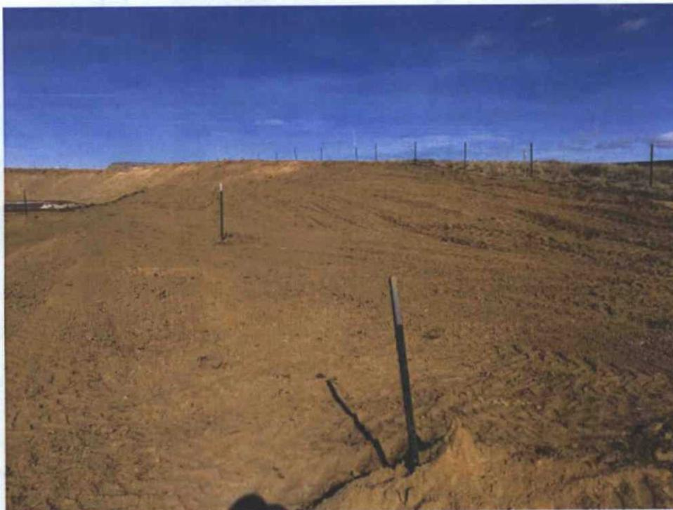
Figure 6: T-posts mark the corners of the cuttings trench. Surface is graded level.
