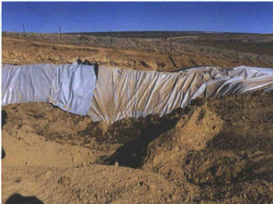
Figure2: Mixing the drill cuttings with clean soil from trench excavation. Stabilization was achieved at a ratio of 1 (clean): 1 (cuttings).
