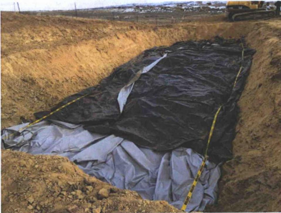
Figure 5: Stabilized cuttings "burrito wrapped" prior to placement of 4 feet soil cap.
