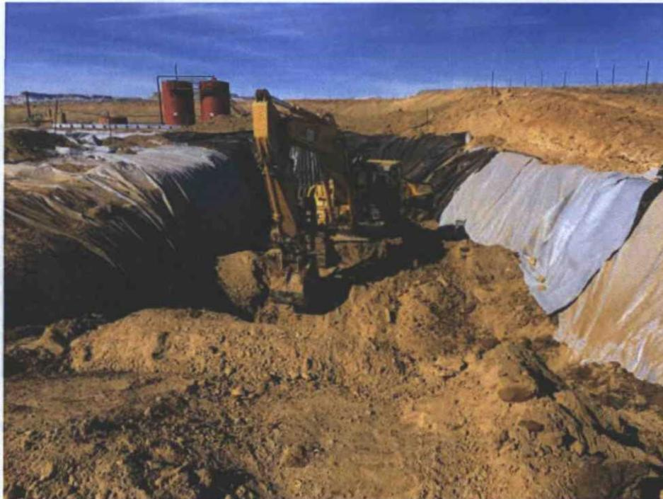
Figure 1: Mixing the cuttings in the lined burial trench.
