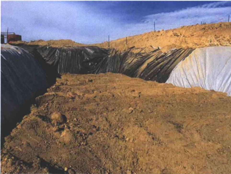
Figure 3: Final mixed cutting in cuttings trench. The trench is lined with a 20-mil string reinforced LLDPE liner.
