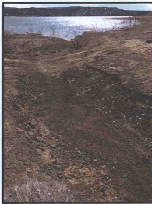
Photo of the lake inlet after removal of liner and berms and the application and raking of gypsum.
