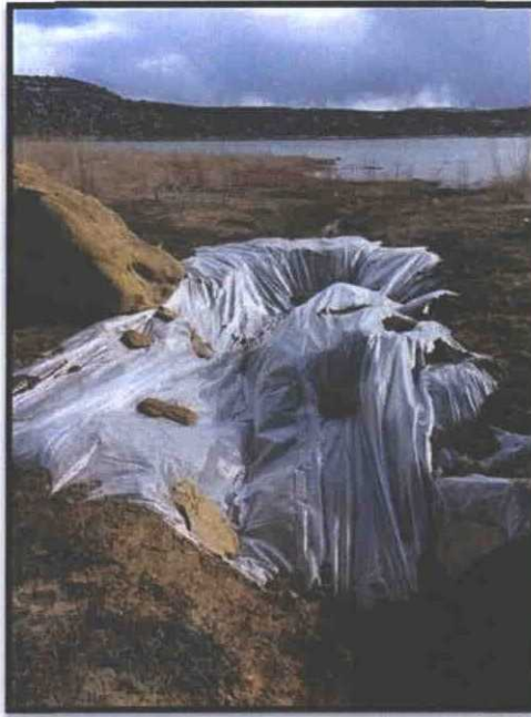
Photo of the liner and berms installed at the lake inlet. The liner and berms were removed on 2/29/2016.
