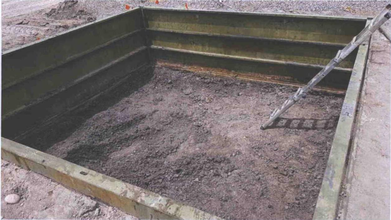
Photograph 1. View facing southwest: final excavation following removal of hydrocarbon impacted soils.
