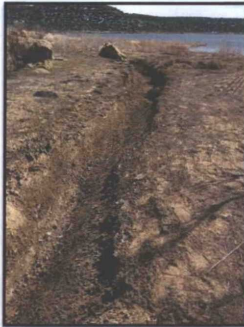
Photo of the lake inlet channel after the application of gypsum.
