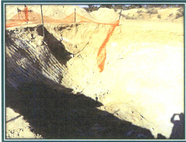
Picture 1: View of Excavation Prior to Potassium Permanganate Application (View to Southwest)
