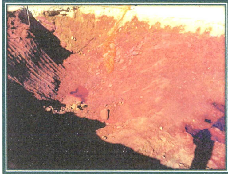
Picture 5: View of Excavation Subsequent to Potassium Permanganate Application (View to Southwest)
