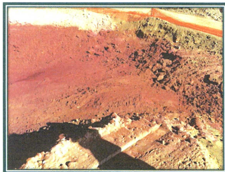
Picture 6: View of Excavation Subsequent of Potassium Permanganate Application (View to East)
