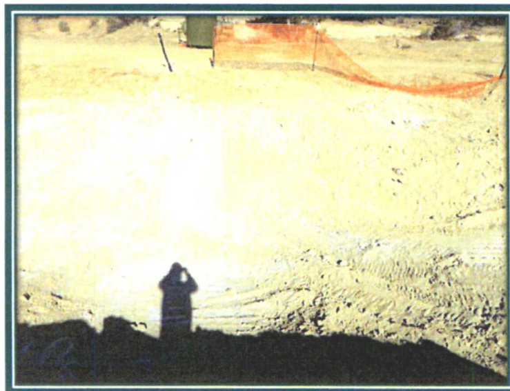
Picture 2: View of Excavation Prior to Potassium Permanganate Application (View to West)
