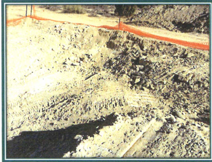
Picture 3: View of Excavation Prior to Potassium Permanganate Application (View to North)
