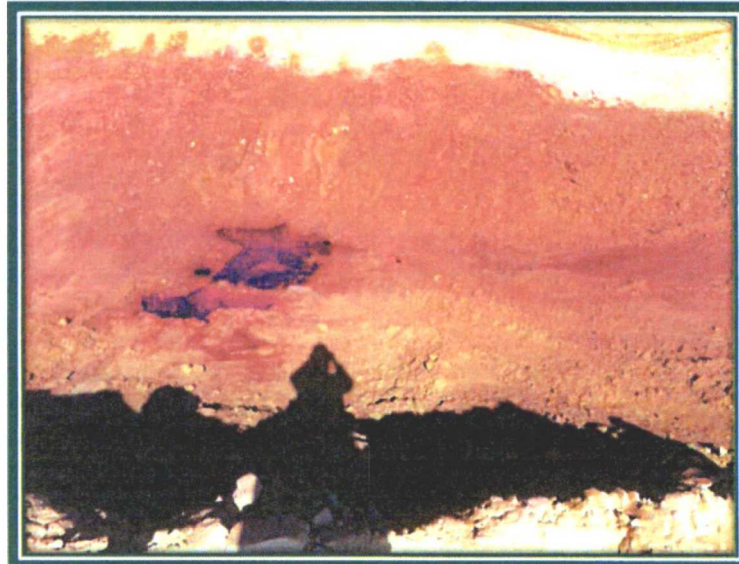
Picture 4: View of West Wall and Bottom North Subsequent of Potassium Permanganate Application
