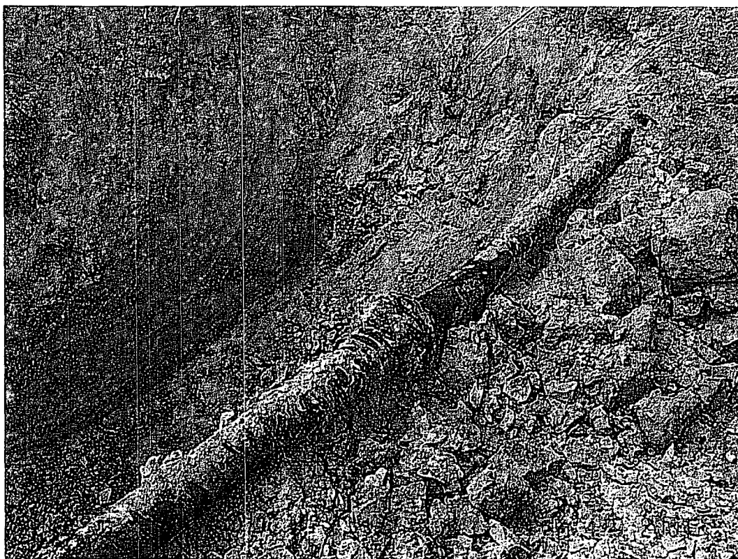
JC4-830 View of flange on 6" dia. wrapped steel pipeline at west end of excavation.
