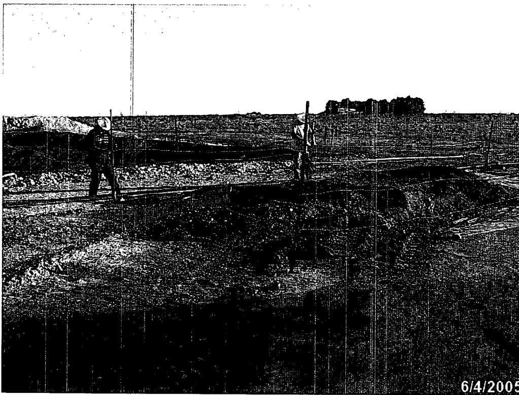
Photograph #4: Saturated soil stockpiled on plastic and fenced.
