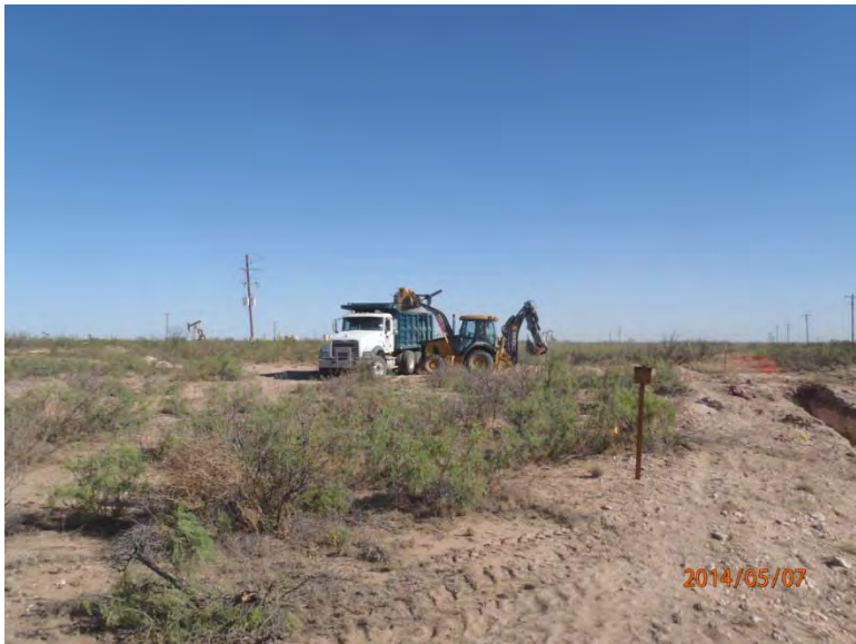
Exporting soil, facing northwest
