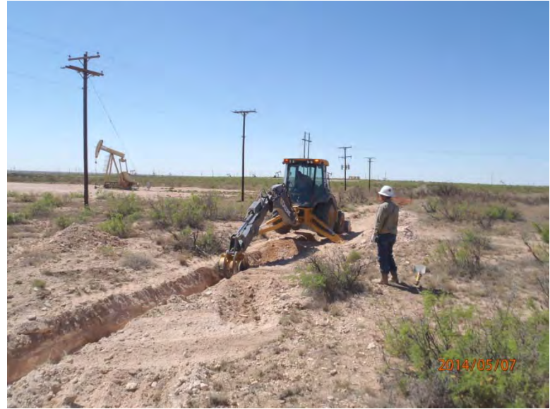
Excavating release, facing southeast
