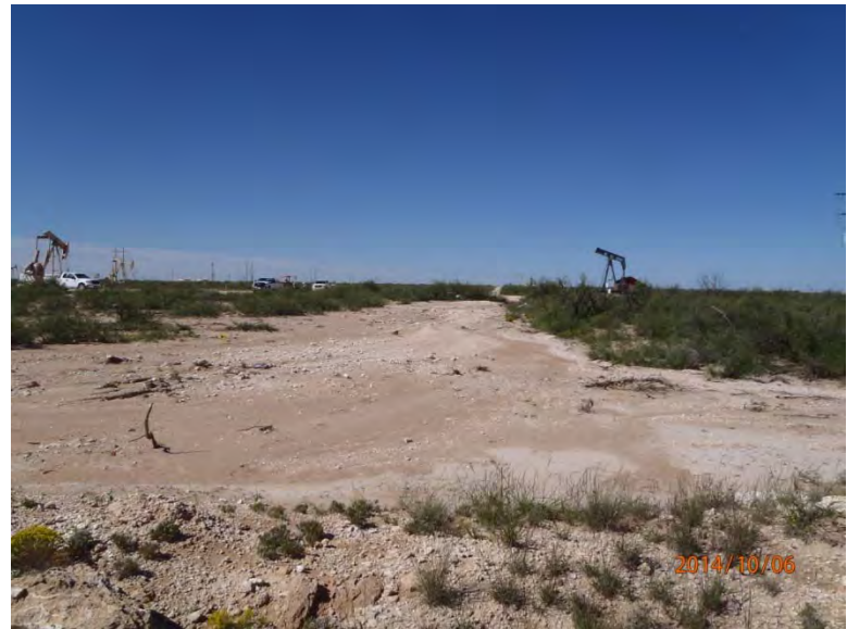
Site backfilled, facing west
