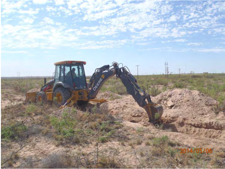
Excavating release, facing southeast
