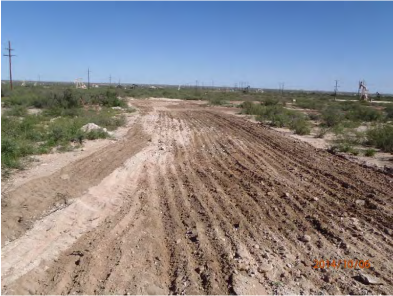
Final photo, facing east
