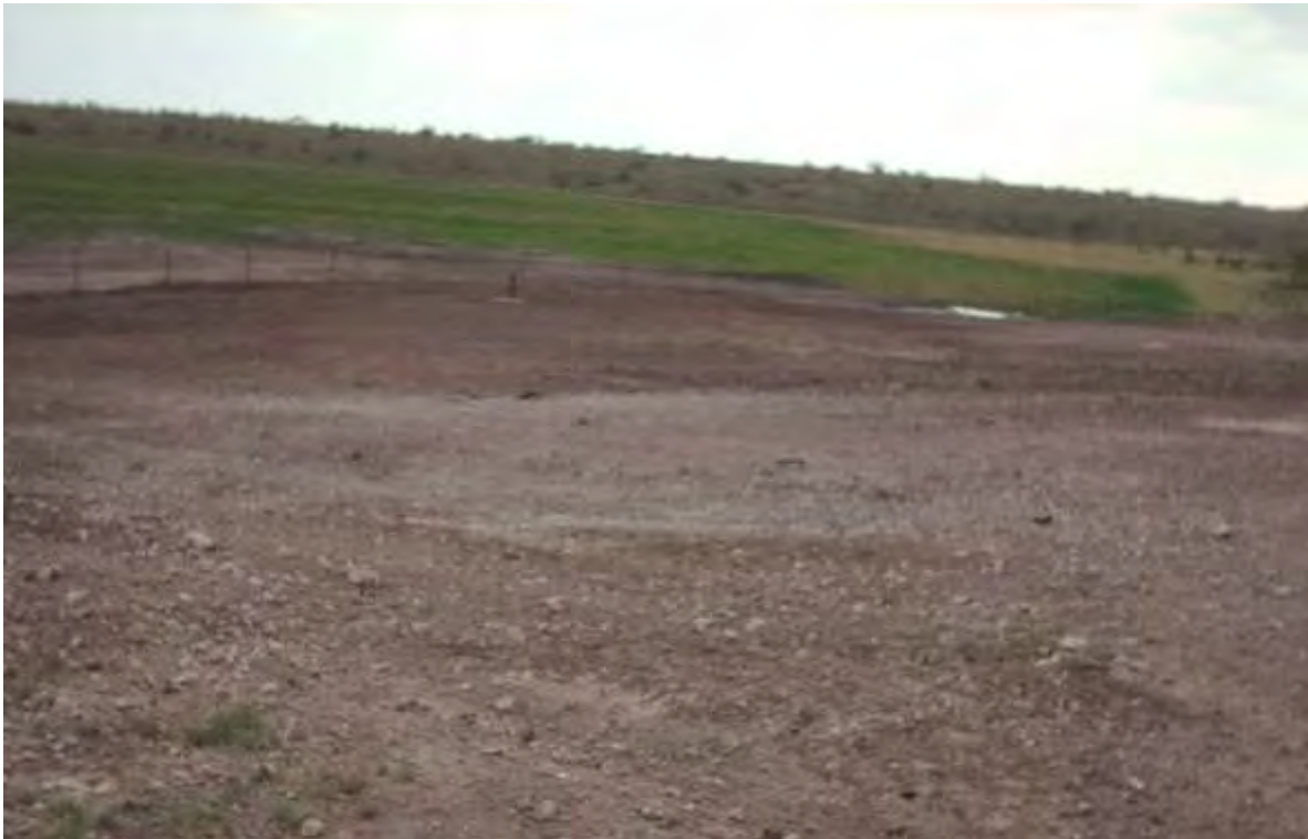
EK Queen Pearce 6-Inch – Backfilled Excavation (Following 2009 Seeding Event; Monitor Well MW-3 Visible in Background)
