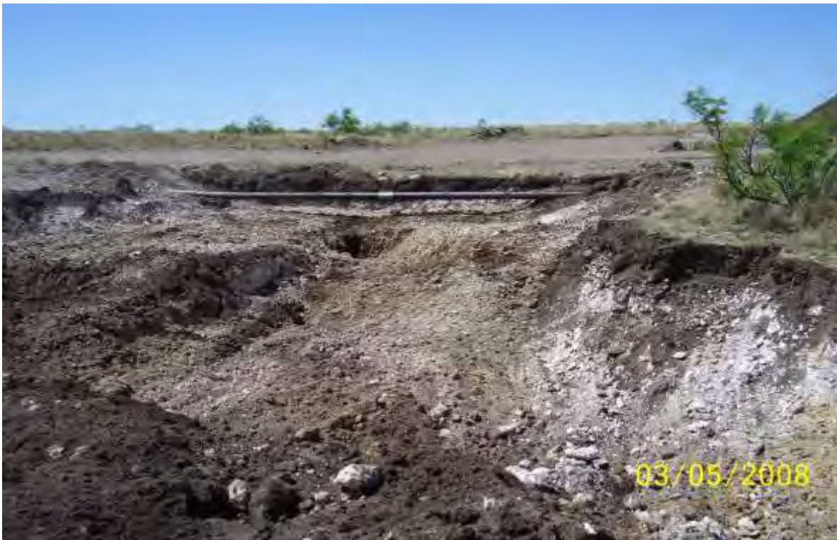
EK Queen Pearce 6-Inch – Excavation (Looking North)
