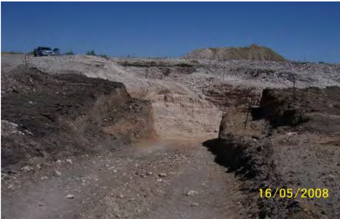
EK Queen Pearce 6-Inch – Excavation (Looking North)
