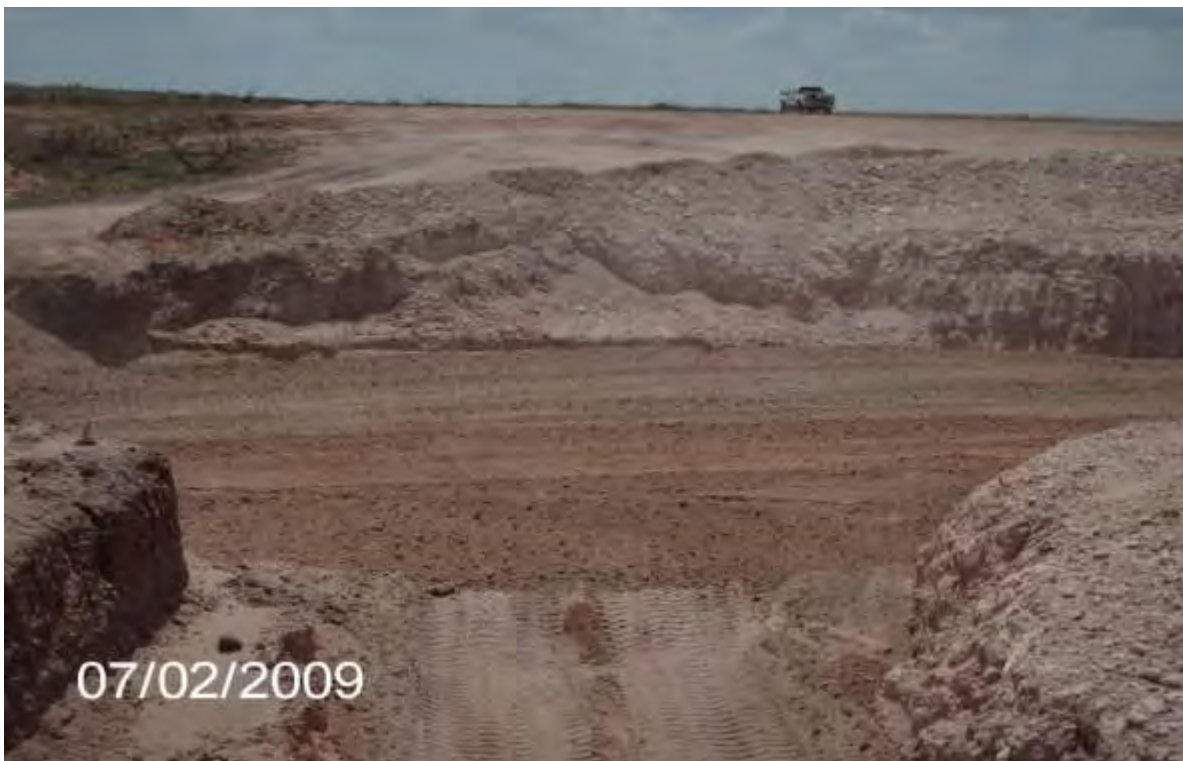
EK Queen Pearce 6-Inch - Backfilling
