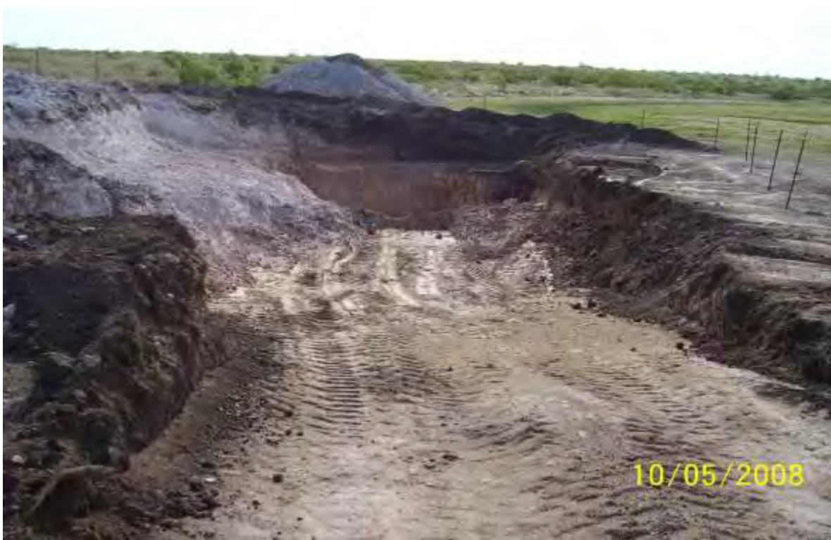
EK Queen Pearce 6-Inch – Excavation (Looking Southeast)
