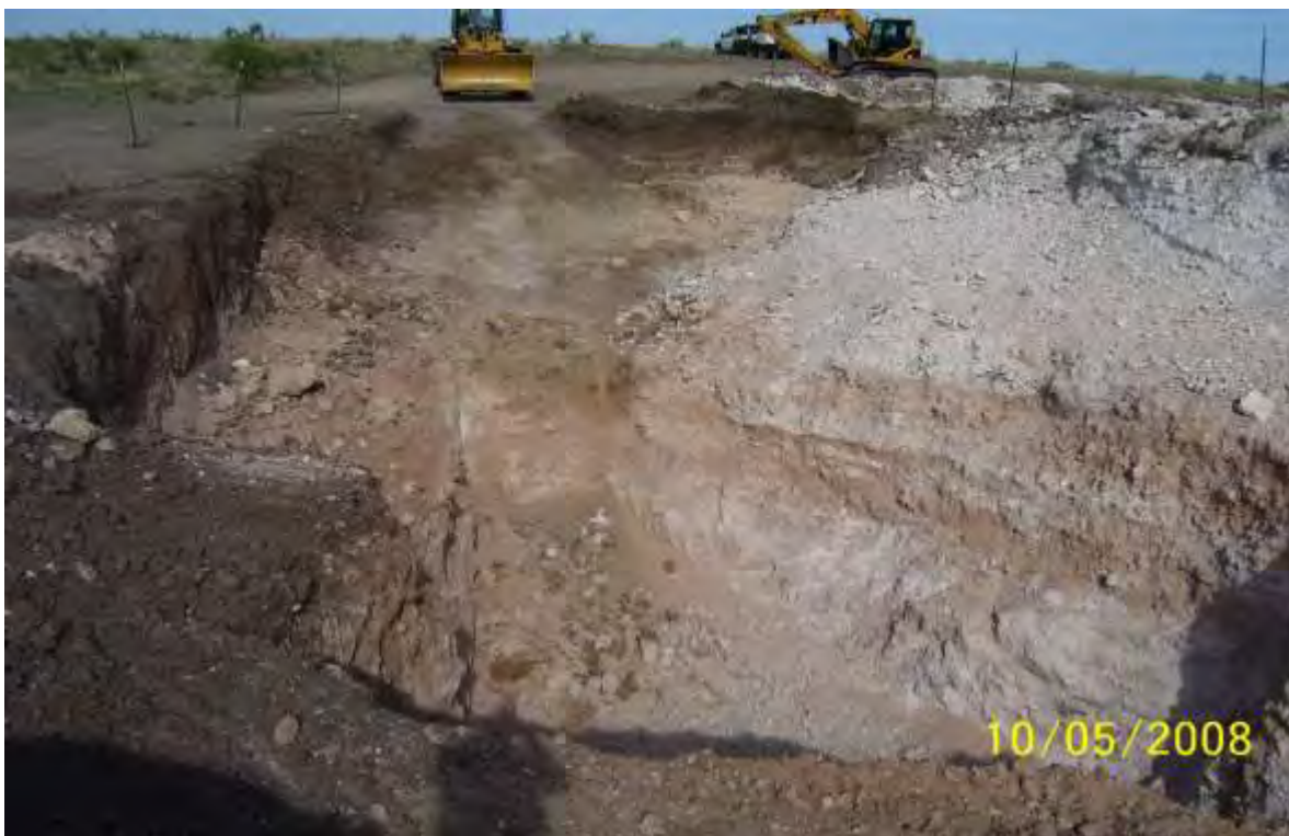
EK Queen Pearce 6-Inch – Excavation
