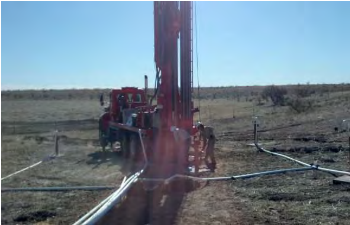
EK Queen Pearce 6-Inch – Advancement of Soil Boring SB-8
