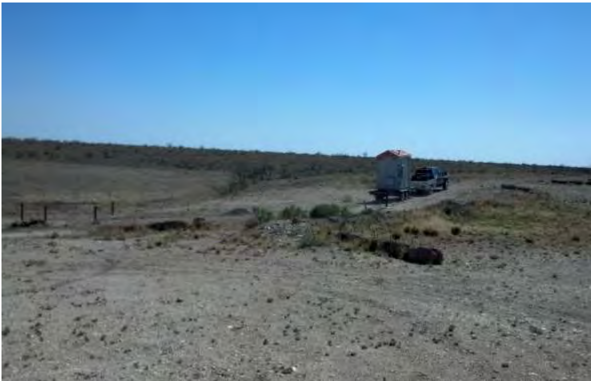
EK Queen Pearce 6-Inch – SVE System Removal
