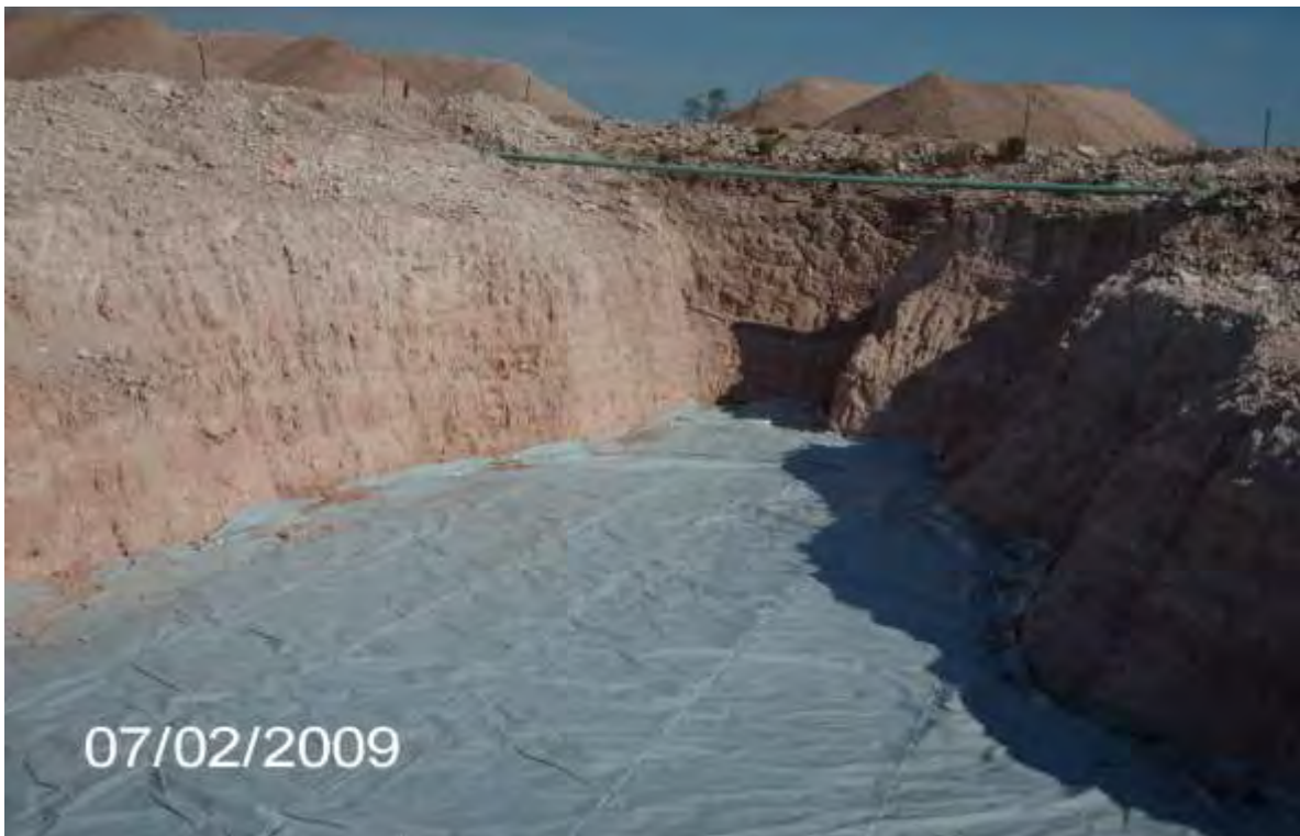
EK Queen Pearce 6-Inch - Liner Installation
