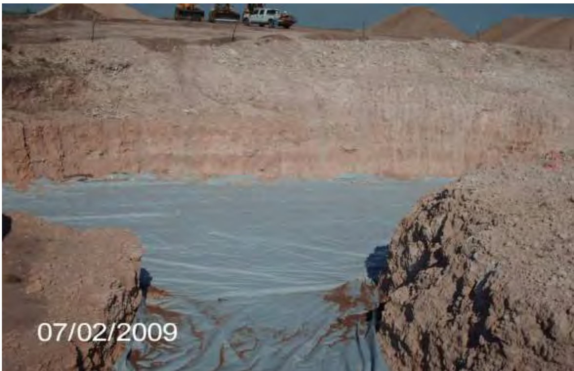
EK Queen Pearce 6-Inch – Liner Installation
