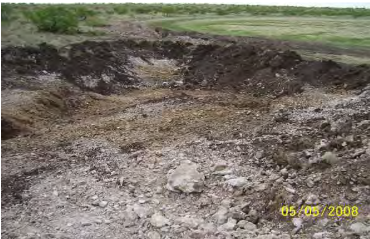
EK Queen Pearce 6-Inch – Excavation (Looking Southeast)
