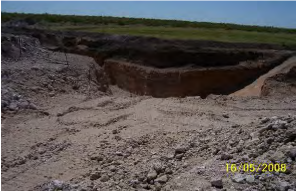
EK Queen Pearce 6-Inch – Excavation (Looking South)
