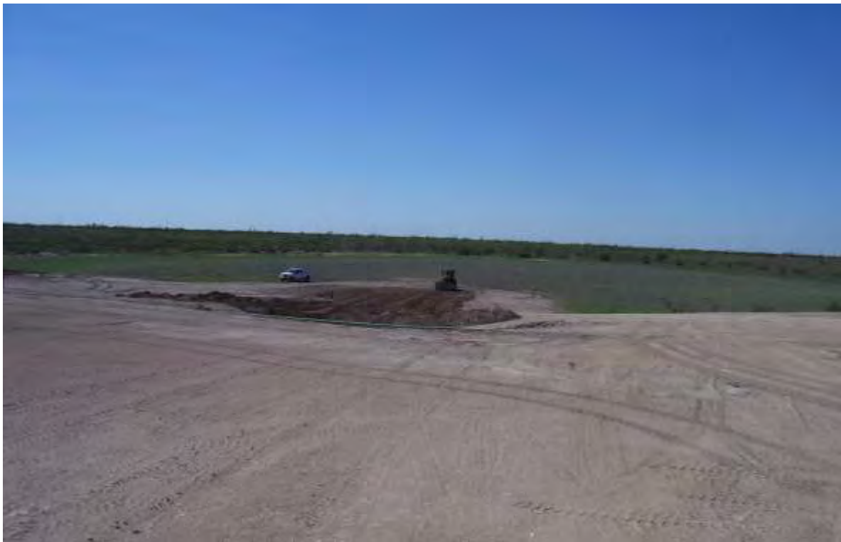
EK Queen Pearce 6-Inch – Backfilling (Near Completion, Looking South)
