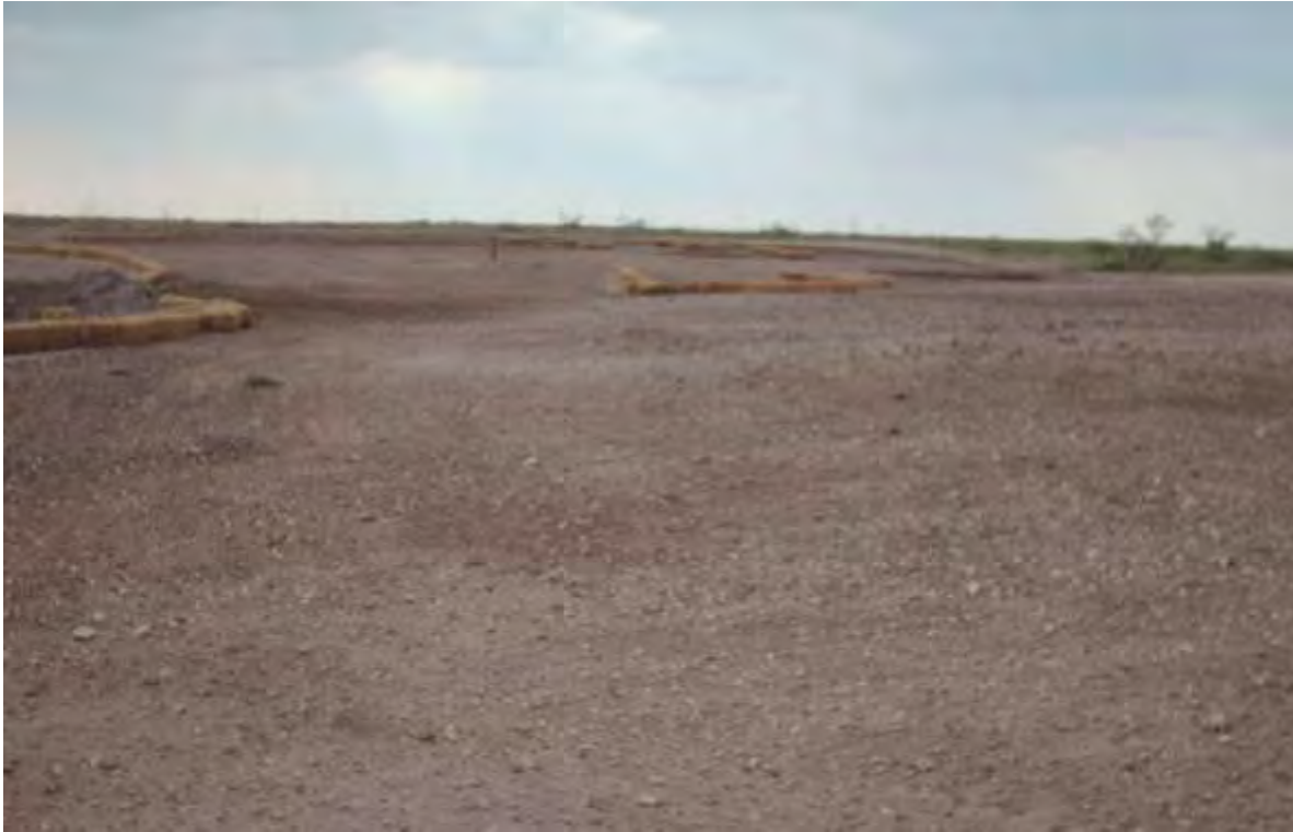
EK Queen Pearce 6-Inch – Backfilled Excavation (Following Seeding; Monitor Well MW-1 & Erosion Control System Visible in Background)
