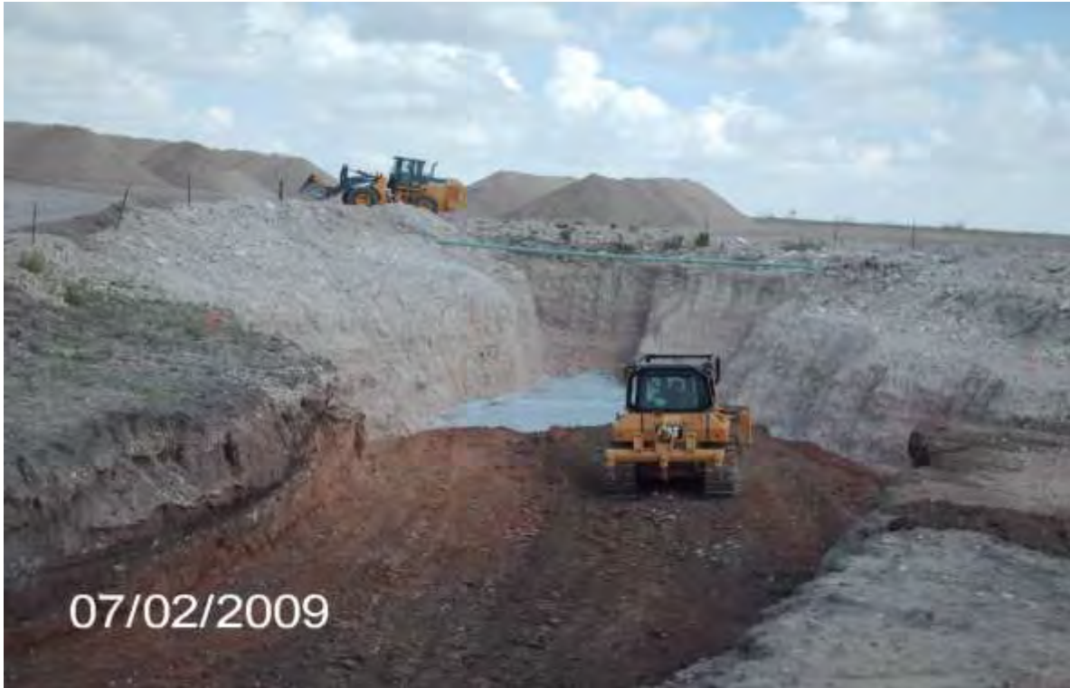
EK Queen Pearce 6-Inch – Pad Sand Installation & Backfilling
