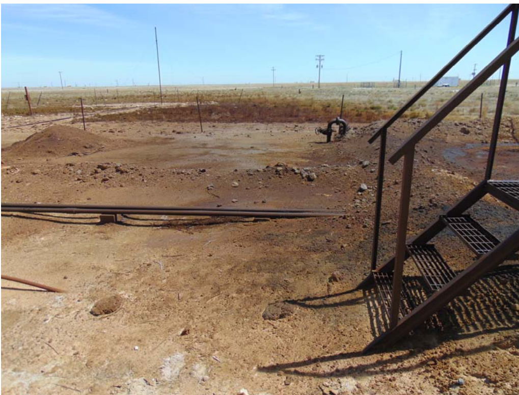
Photograph #2- Overspray area on northeast end of release
