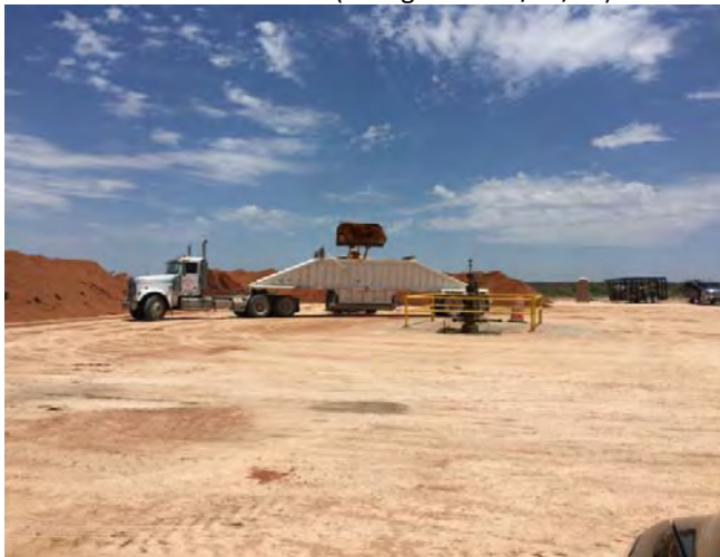
Loading belly dump with ~20 yd 3 of chloride-impacted soil for disposal at Lea Land landfill.
