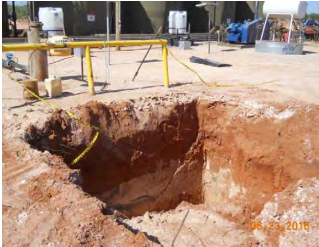
DP-1 area at release source (loading valve) excavated to depth of 8' bgs.
