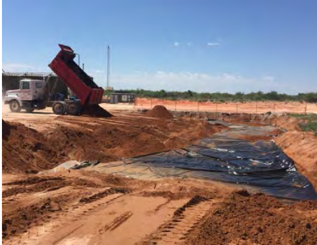
DP-5 and DP-6 areas backfilled to 4' bgs with 20-mil reinforced liner and backfilling activities (facing south).
