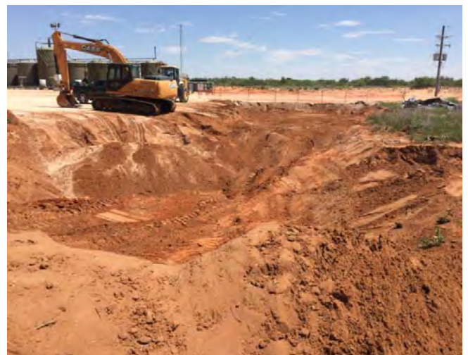
DP-6 area excavated to 8' bgs (facing south on 6/14/16).
