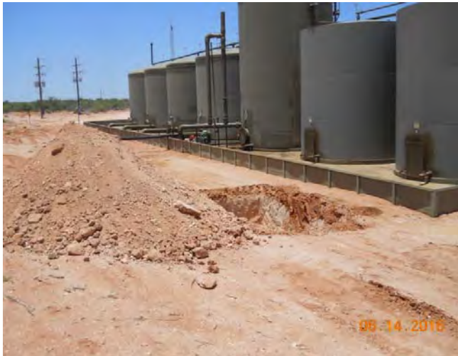
DP-3 area behind southeast corner of tank battery excavated to depth of 8' bgs.
