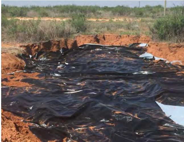
DP-8 area excavated and then backfilled to depth of 4' bgs with 20-mil reinforced liner (facing SW on 6/10/16).
