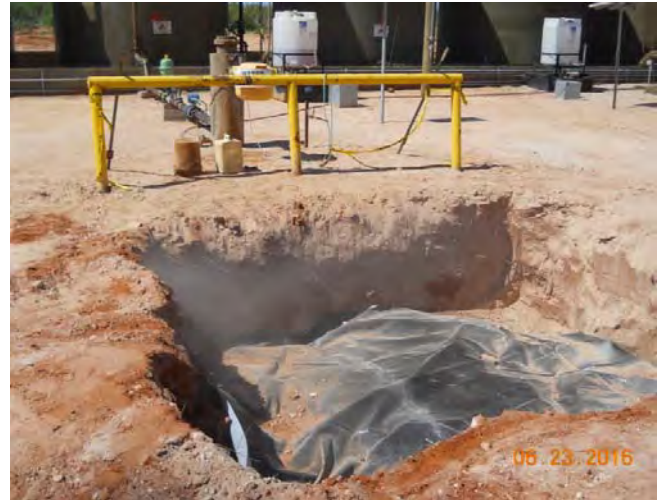
DP-1 area at release source (loading valve) backfilled to depth of 4' bgs with 20-mil reinforced liner.
