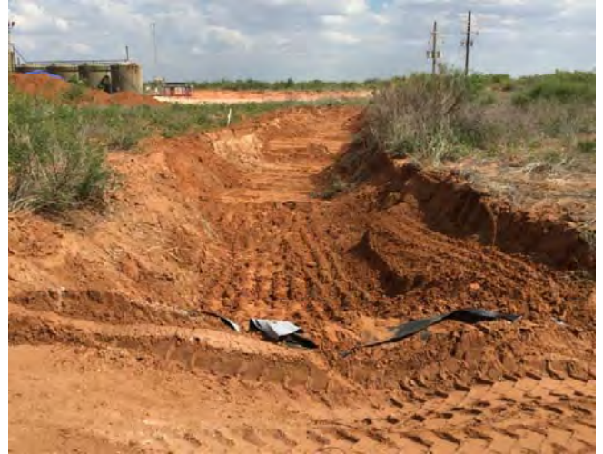
DP-7 area excavated and backfilled to 4' bgs prior to liner installation (facing south).
