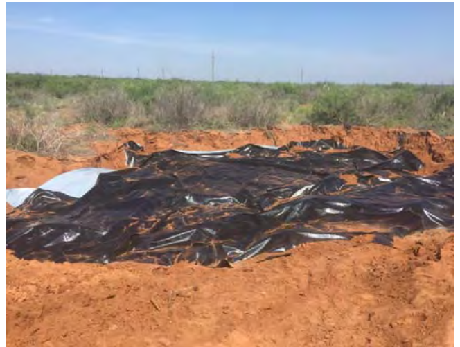
DP-9 area excavated and then backfilled to depth of 4' bgs with 20-mil reinforced liner (facing NW on 6/10/16).
