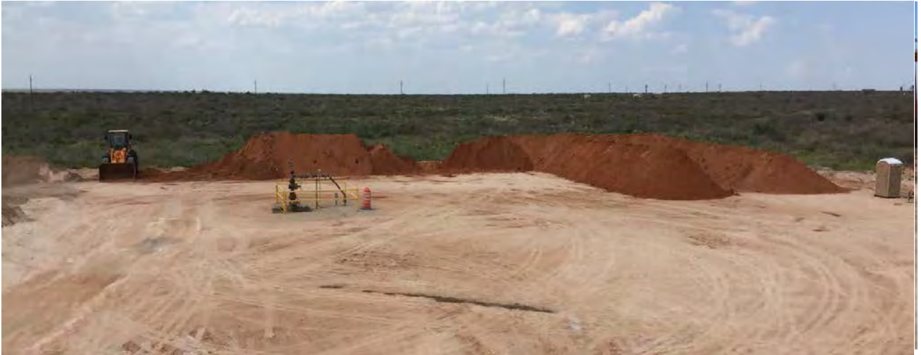
View facing north showing stockpiles of excavated chloride-impacted soil on 6/13/16.
