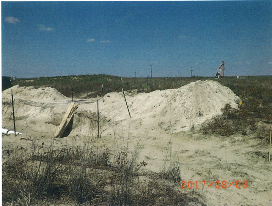
Site Viewing Northeast
