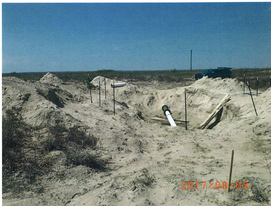
Site Viewing North
