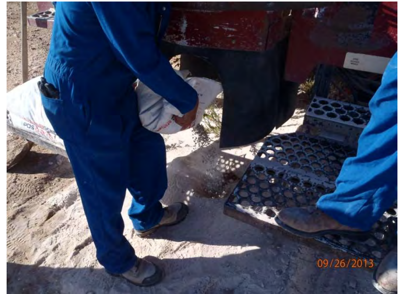
Plug SB-4 in total with bentonite
