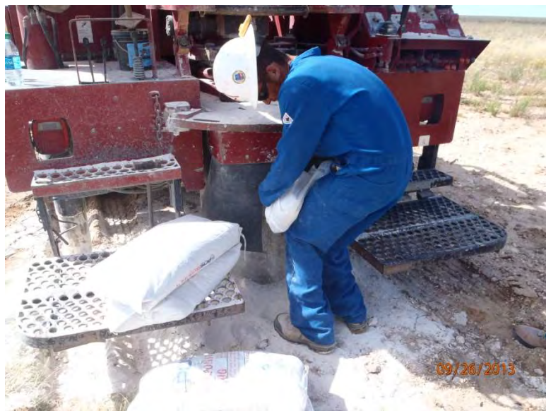
Plugging SB-5 in total with bentonite
