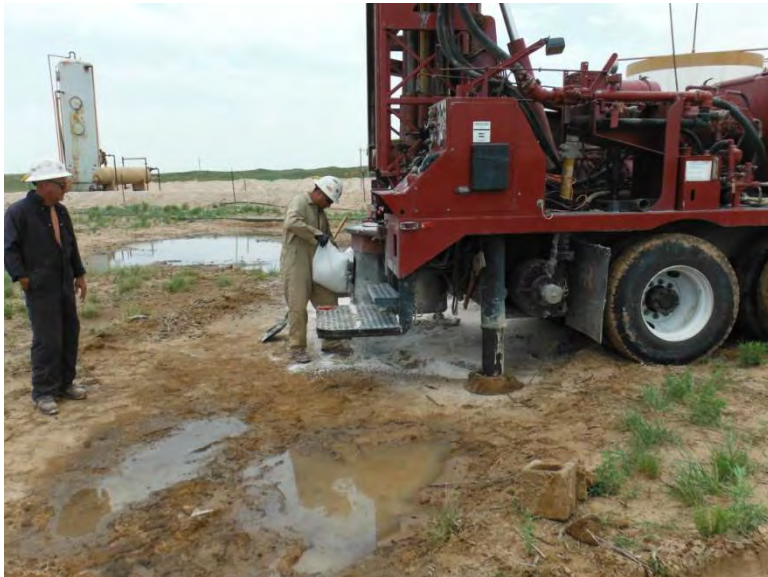
Plugging SB-3 in total with bentonite
