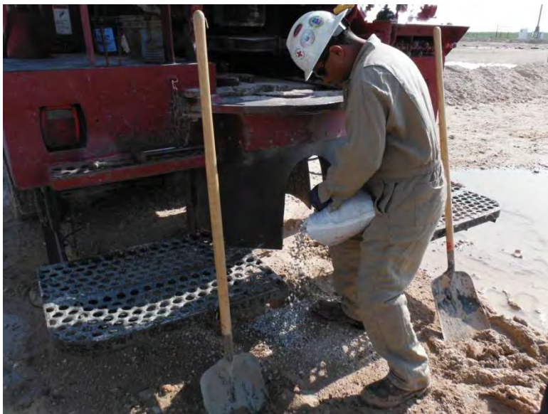
Plugging SB-1 in total with bentonite
