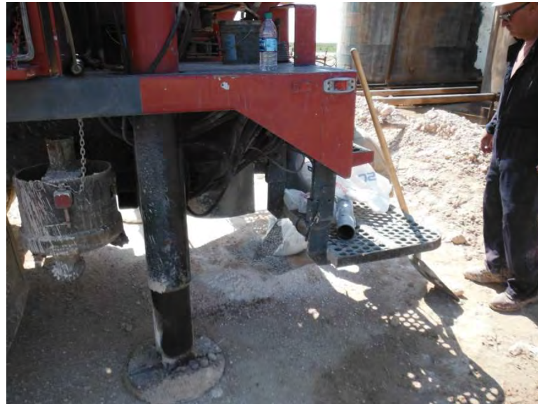
Plugging SB-2 in total with bentonite
