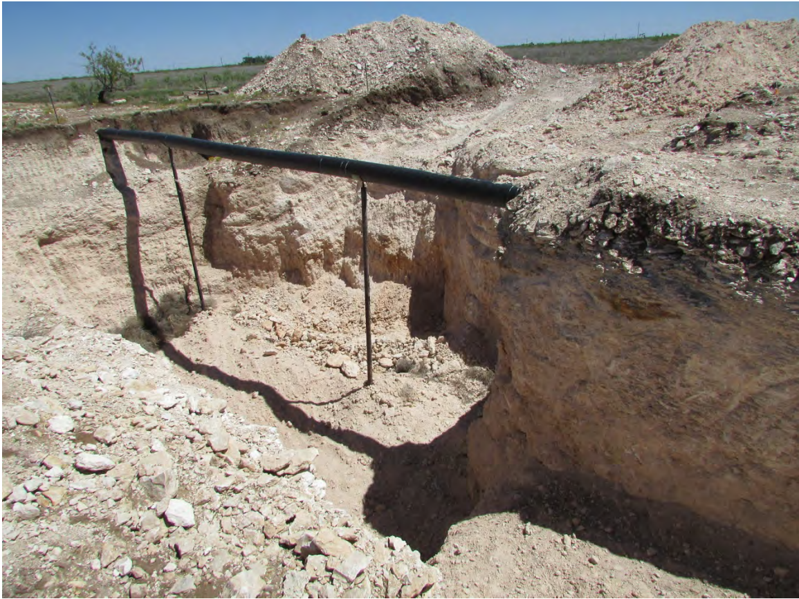
May 10, 2016: Excavation at about 24 feet bgs, showing remaining staining on west wall under pipeline
