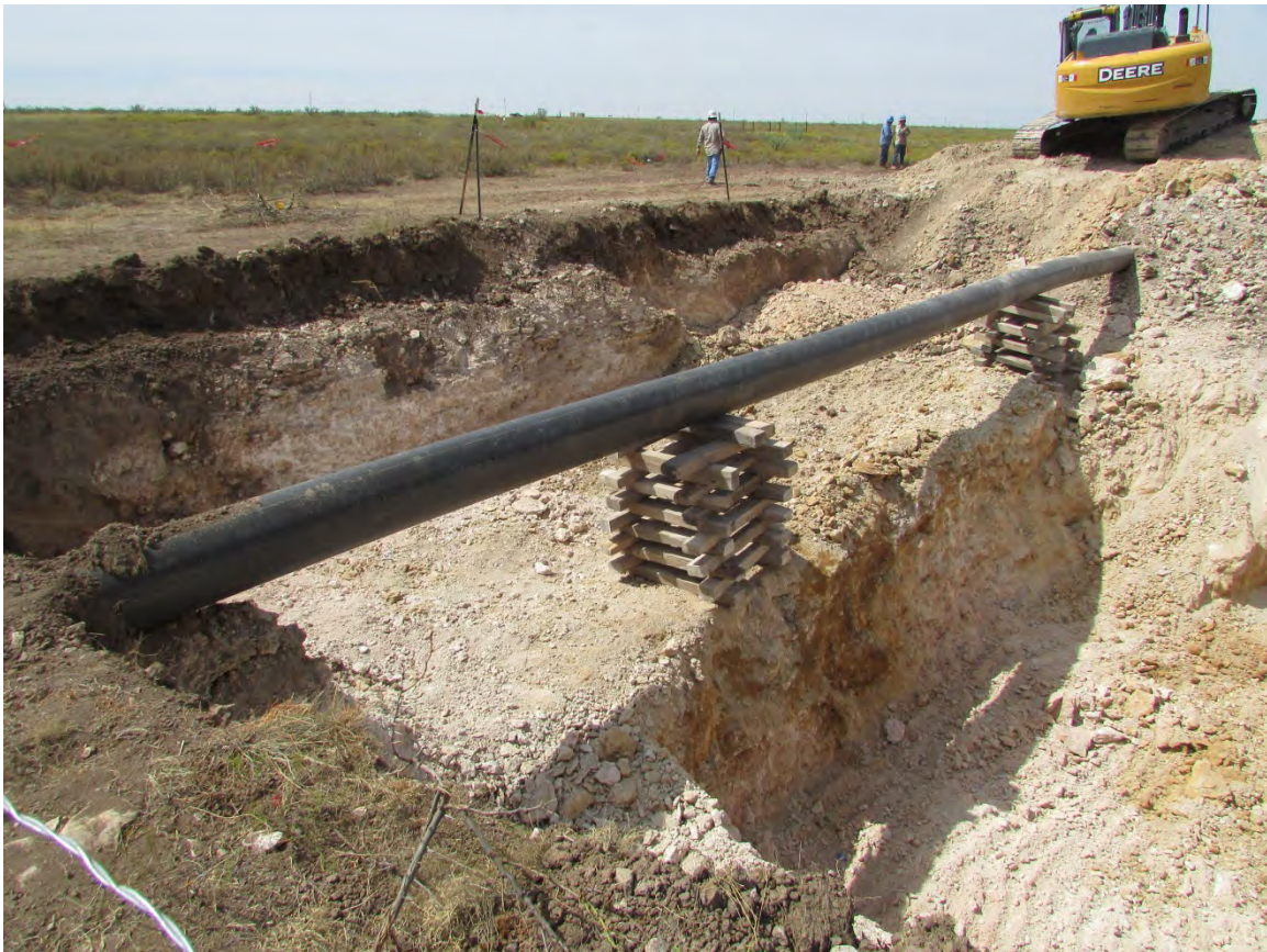
September 21, 2015: Preliminary excavation at about 15 feet bgs, showing staining on south wall
