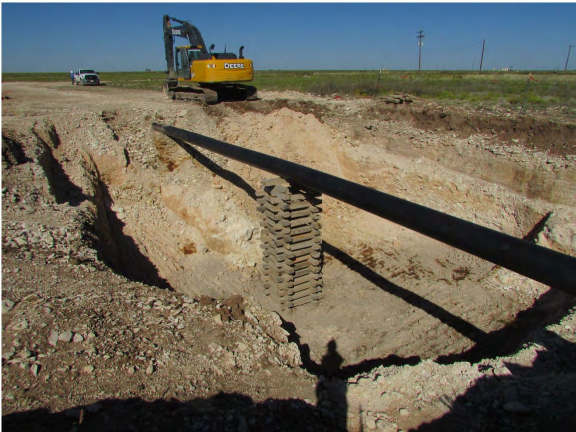
October 13, 2015: Preliminary excavation at about 18 feet bgs, showing staining at bottom and west wall under pipeline
