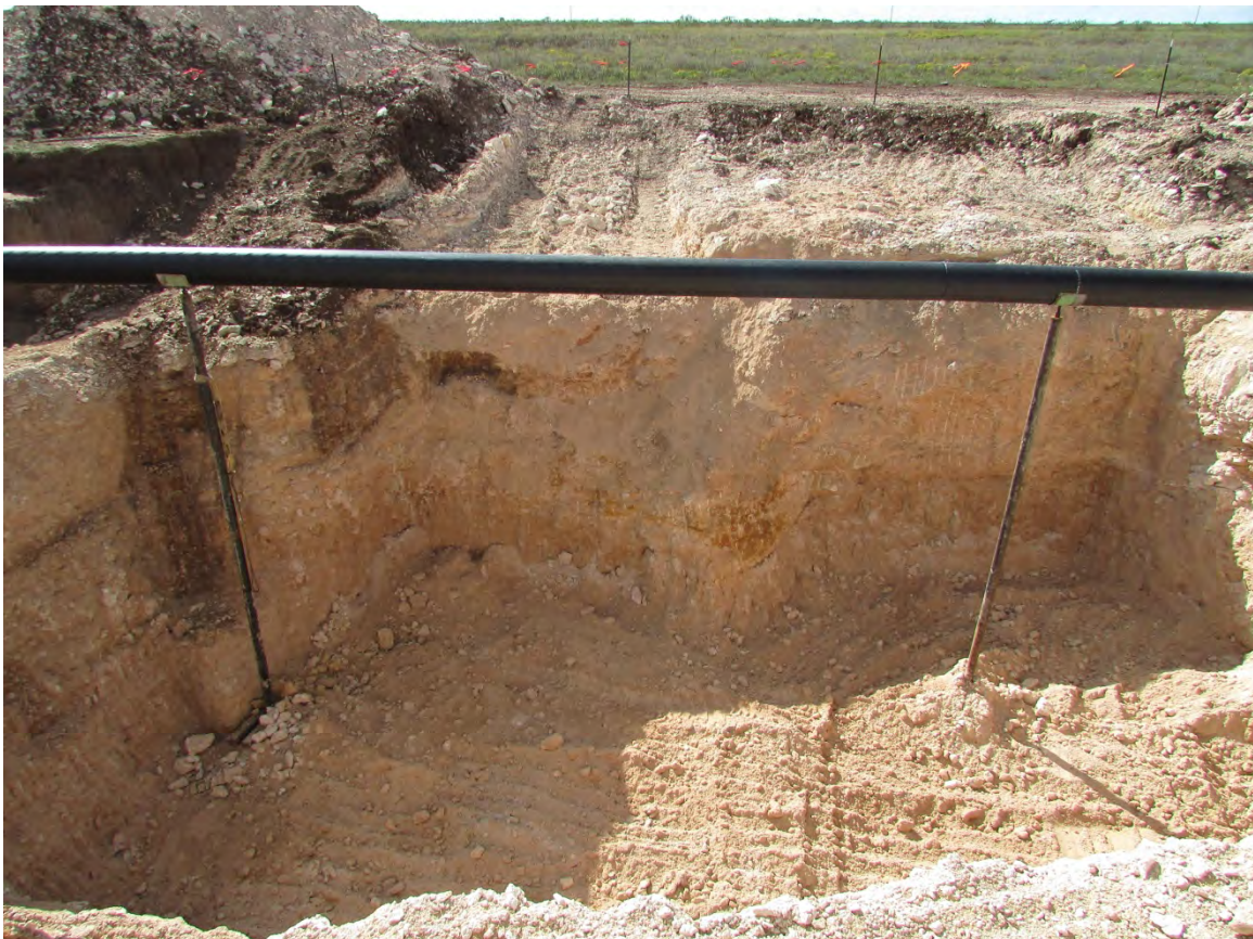
October 30, 2015: Excavation at about 22 feet bgs, facing east, looking at staining on boulder of south wall
