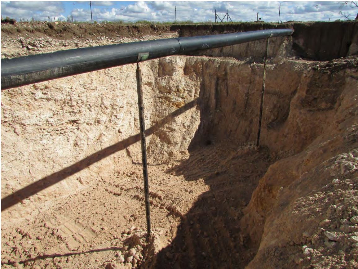
October 30, 2015: Excavation at about 22 feet bgs, facing northeast, looking at staining on NE corner at about 15 feet
