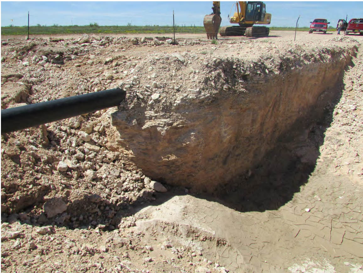
September 19, 2016: Facing Southwest, looking at west wall staining at about 6 feet bgs before removal
