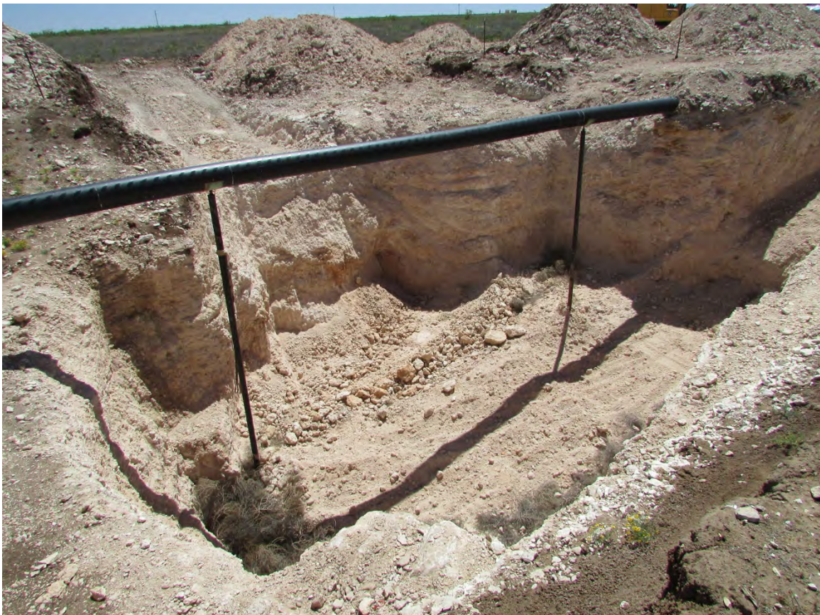
May 10, 2016: Excavation at about 24 feet bgs, showing south wall with stained boulder removed
