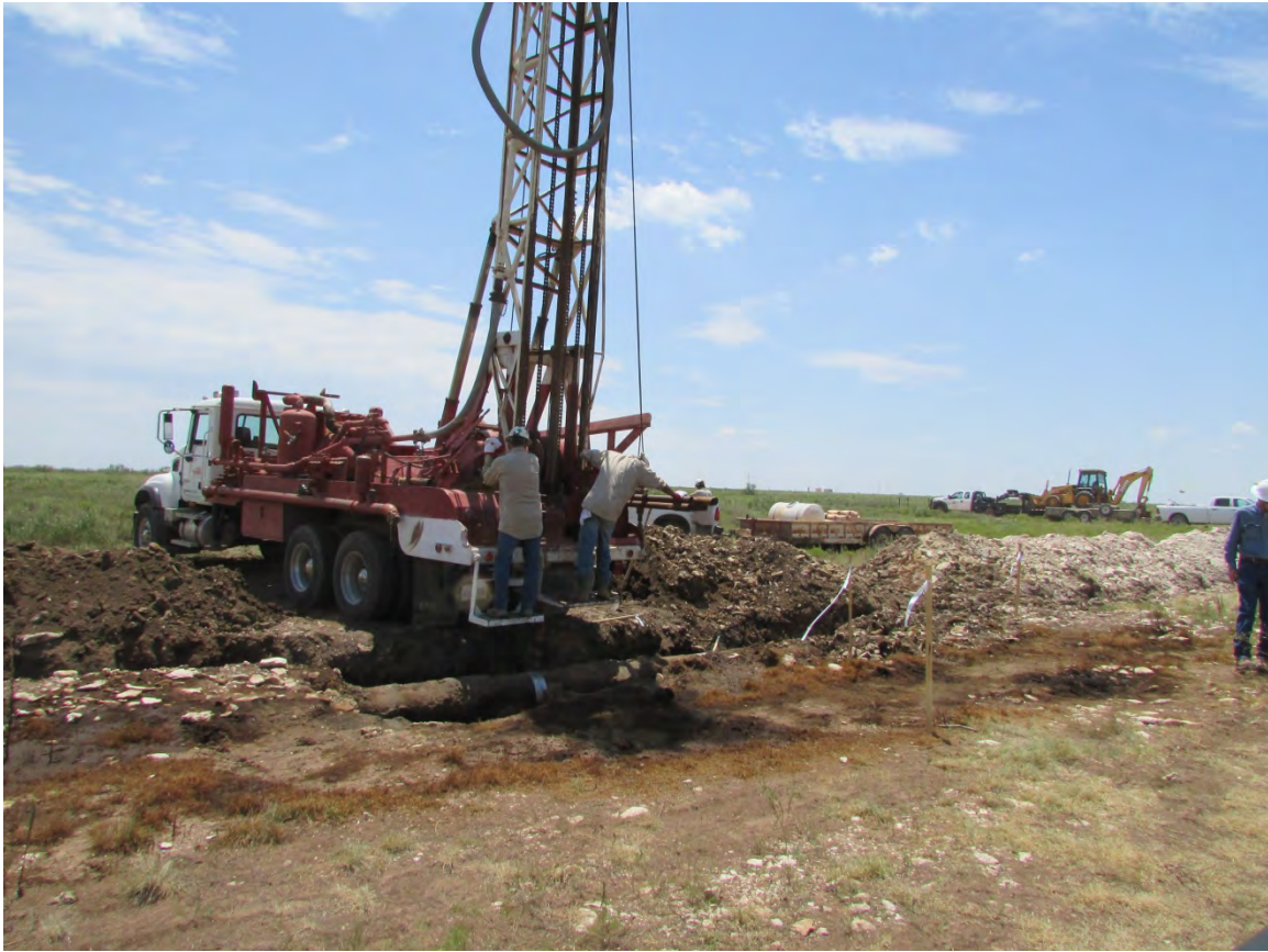
August 3, 2015: Drilling SB-5 soil boring down to 25 feet bgs
