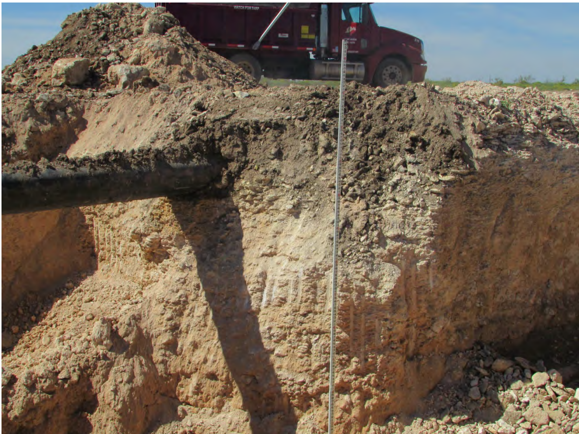
September 20, 2016: Facing Southwest, looking at west wall staining at about 6 feet bgs during soil removal
