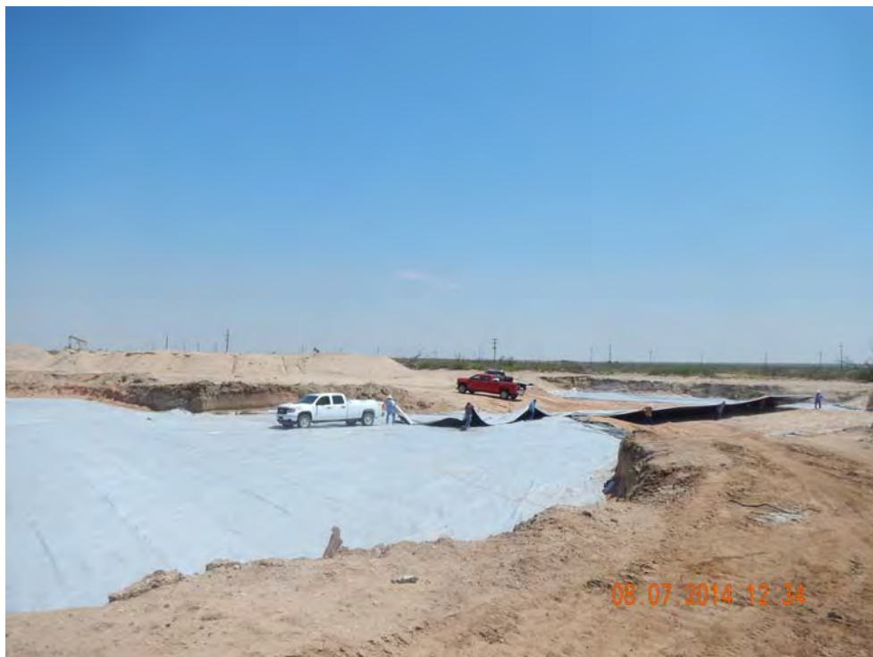
LMPSU Trash Pit, East Excavation Linear Installation, Viewing Northeast
