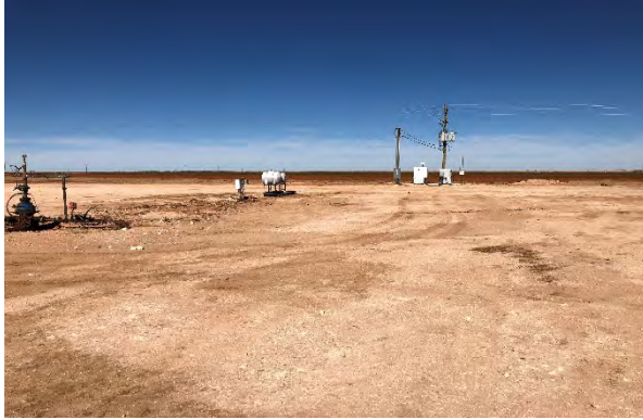
Above: Wellhead facing north, area to be excavated located to the right of the wellhead.
