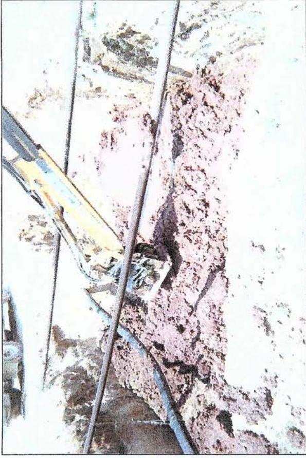
compacting clay
