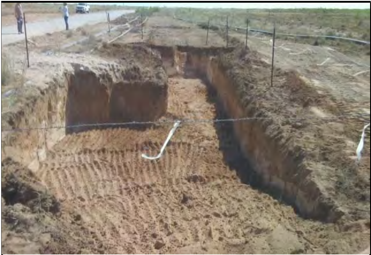
Figure 2 - View of affected area after partial excavation, facing Northeast.
