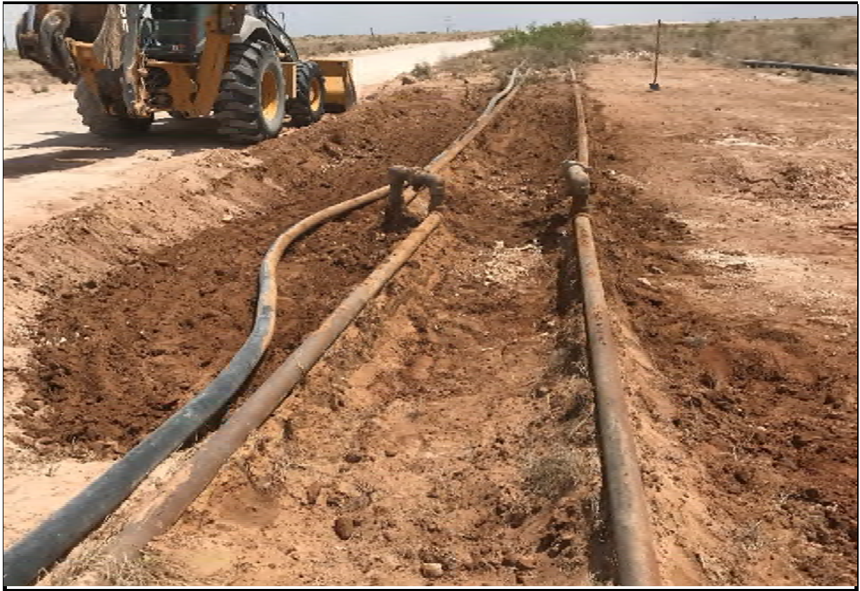
Figure 3 - View of affected area after partial excavation, facing Northeast.
