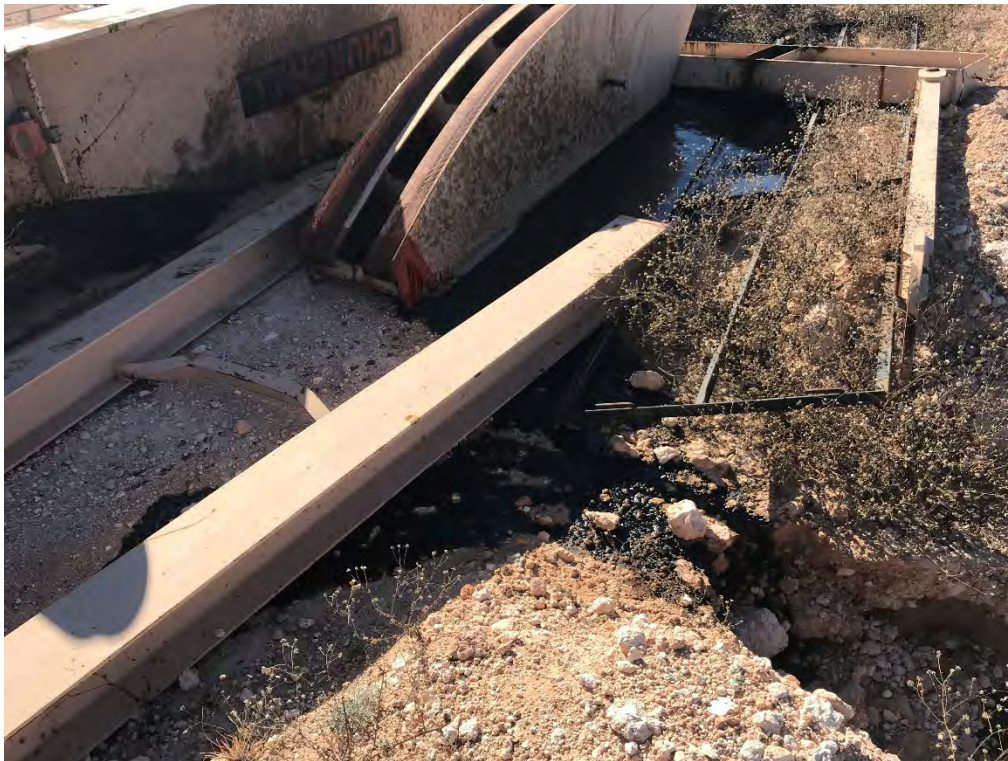
Release (Looking West-Southwest)
