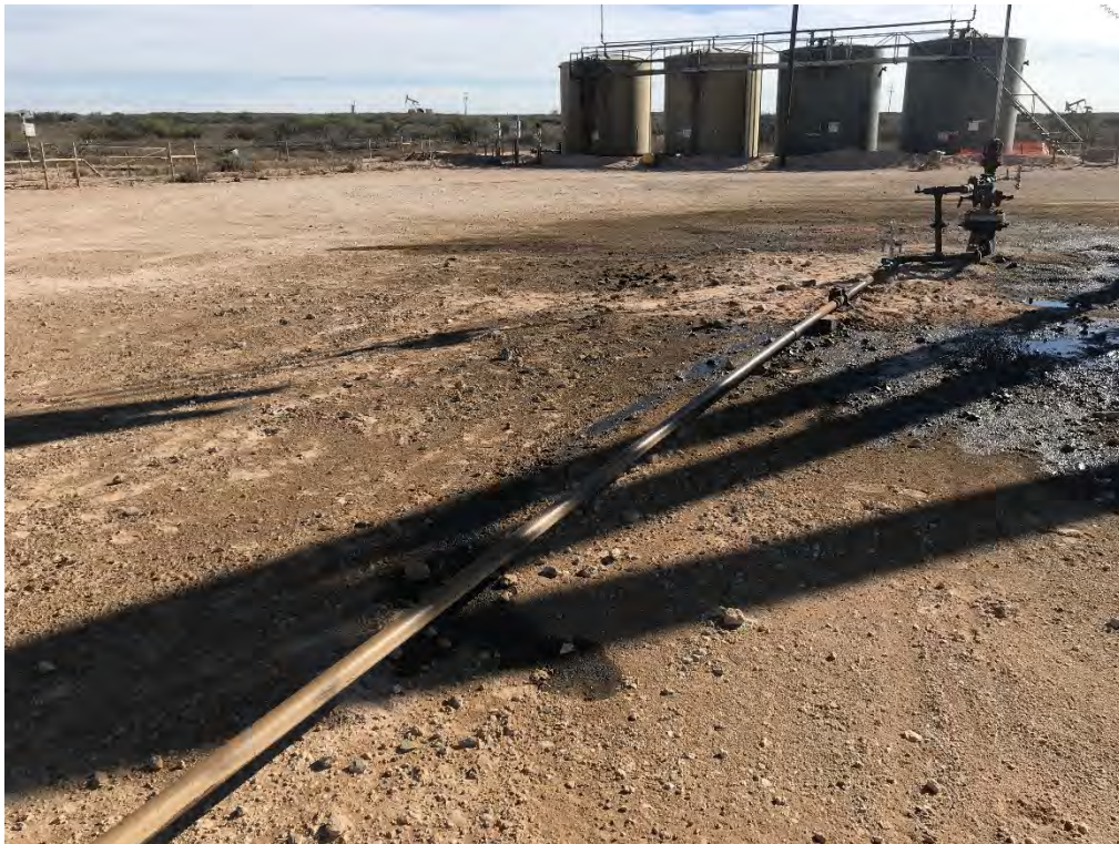
Release (Looking South-Southeast)
