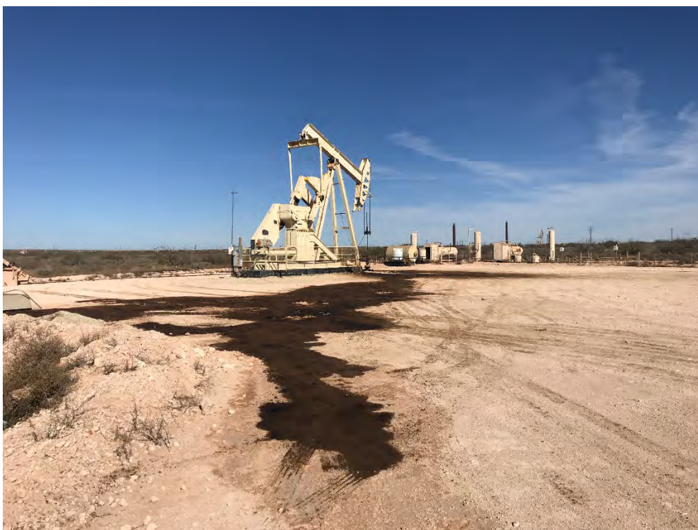
Release (Looking Northeast)
