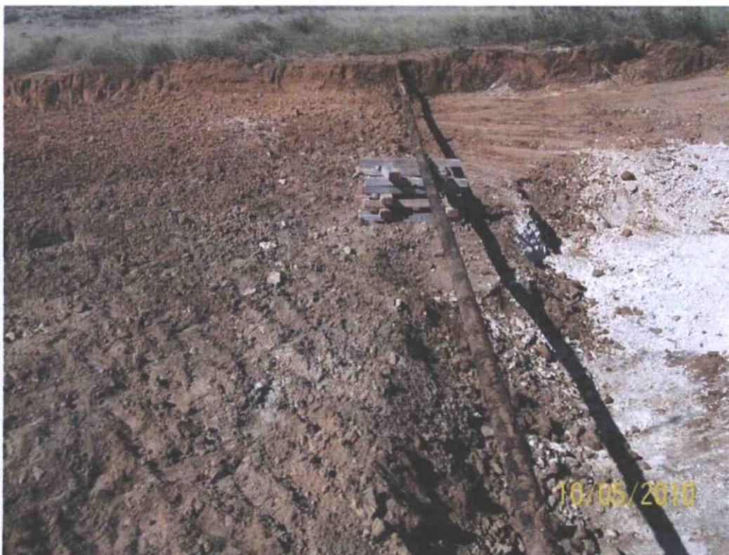
Photograph No. 4 – Looking northerly at initial excavated area and active pipeline supported with wooden brace
