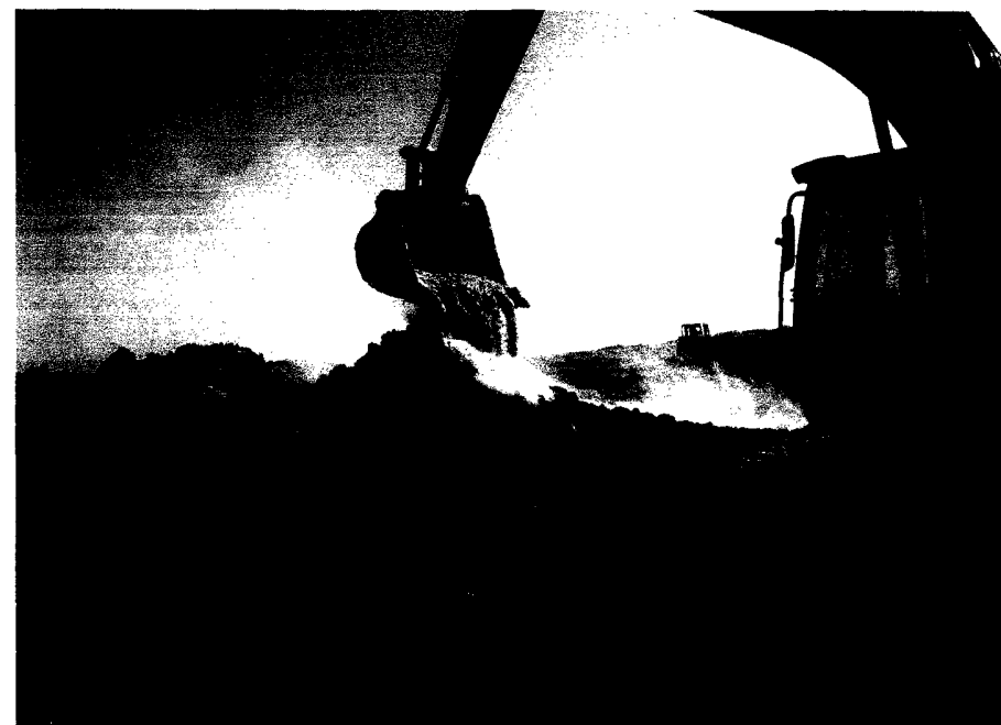
Spreading Elke's solidification material on the mud
