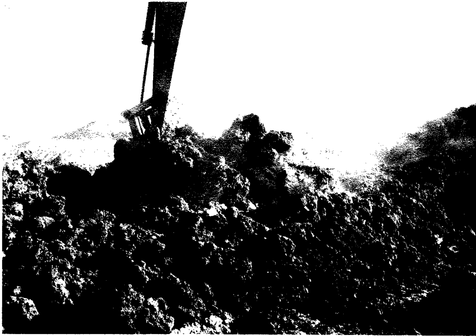
Mixing the solidification material
