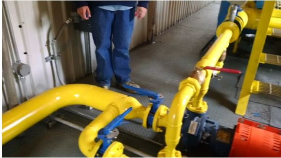
Incoming Tank Effluent Line into Pump House
