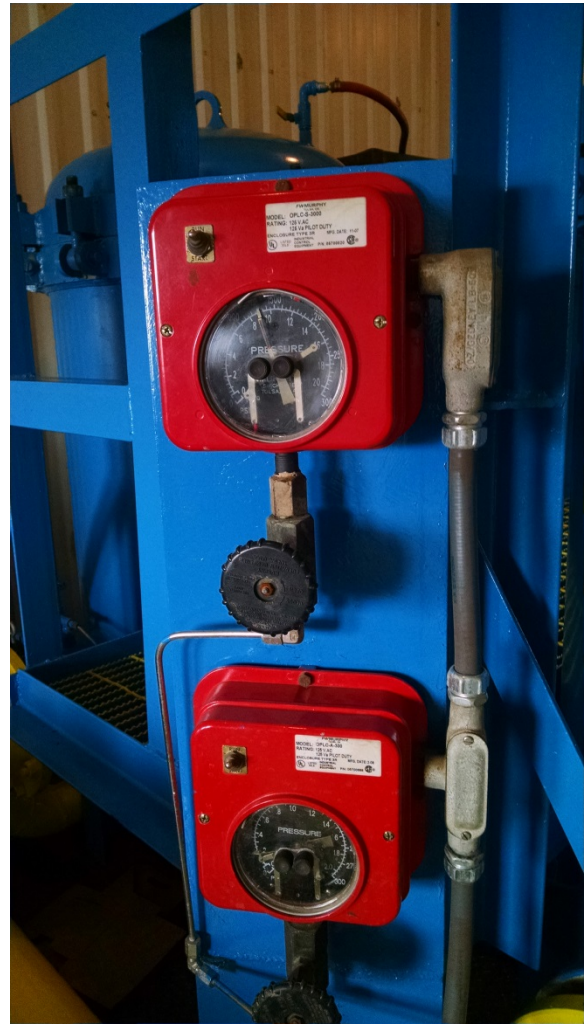
In-line pressure gauges on Filtration Unit
