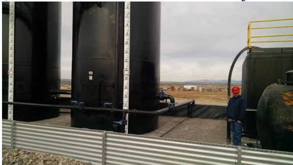
Looking E at sample port at S end of tanks before effluent line to pump house for injection
