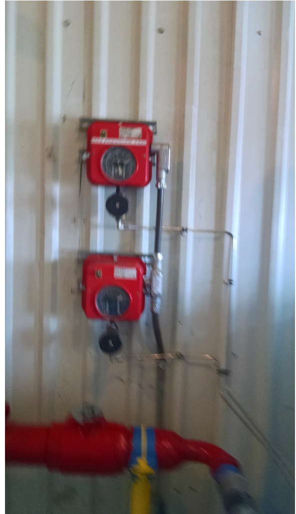
Maximum Surface Injection Pressure with Murphy Auto Shut-Off Switch in Pump House
