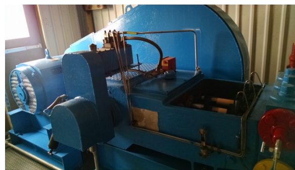
Pump No. 2 in Pump House (two large pumps capable of ~ 155 gpm)
