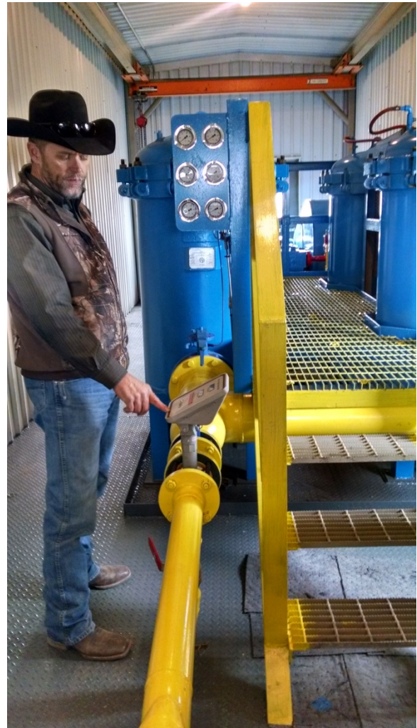
Flow Meter Totalizer with 20micron/5micron Filters in background
