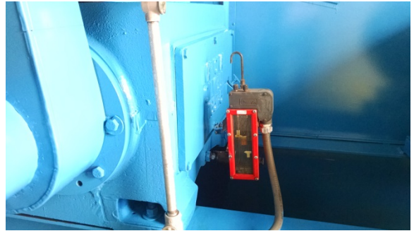
Pump lubrication fluid level meter
