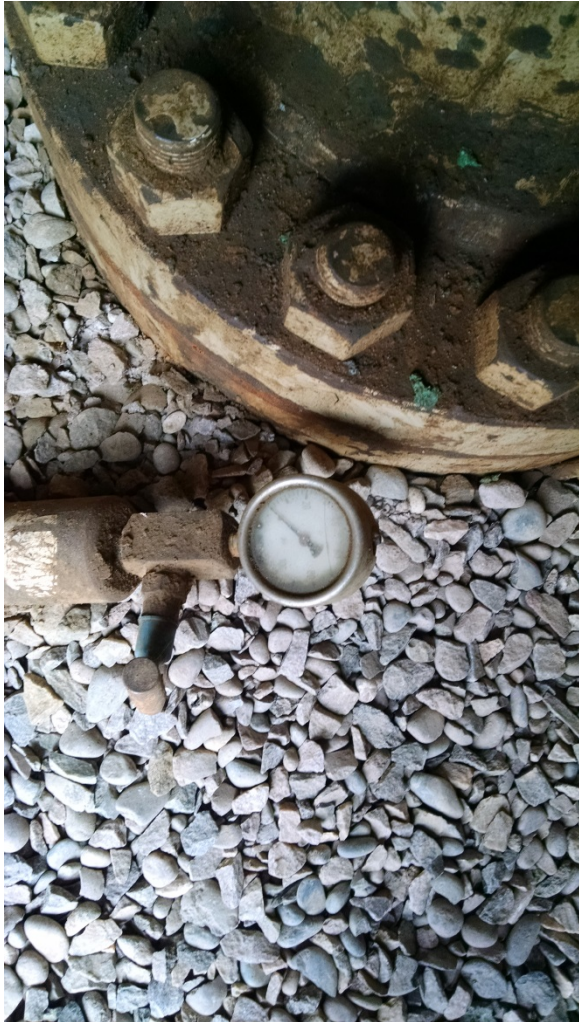
Bradenhead gauge at bottom of injection well
