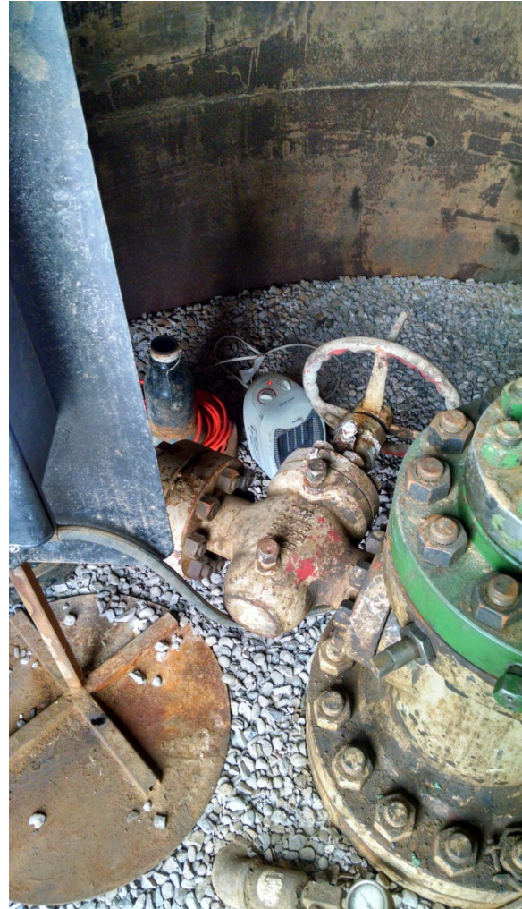
Bradenhead gauge at base of well head
