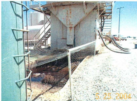
Single lined steel pit. Standing oil and water.
