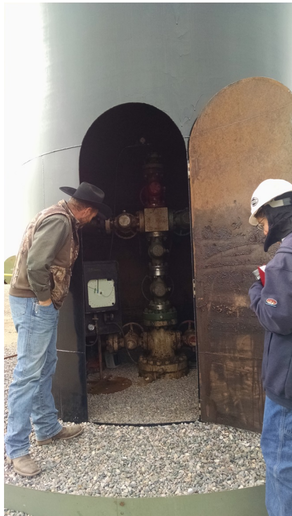
SUNCO WDW No. 1 with Chart Recorder Encapsulated by Modified Tank (no well sign evident)
