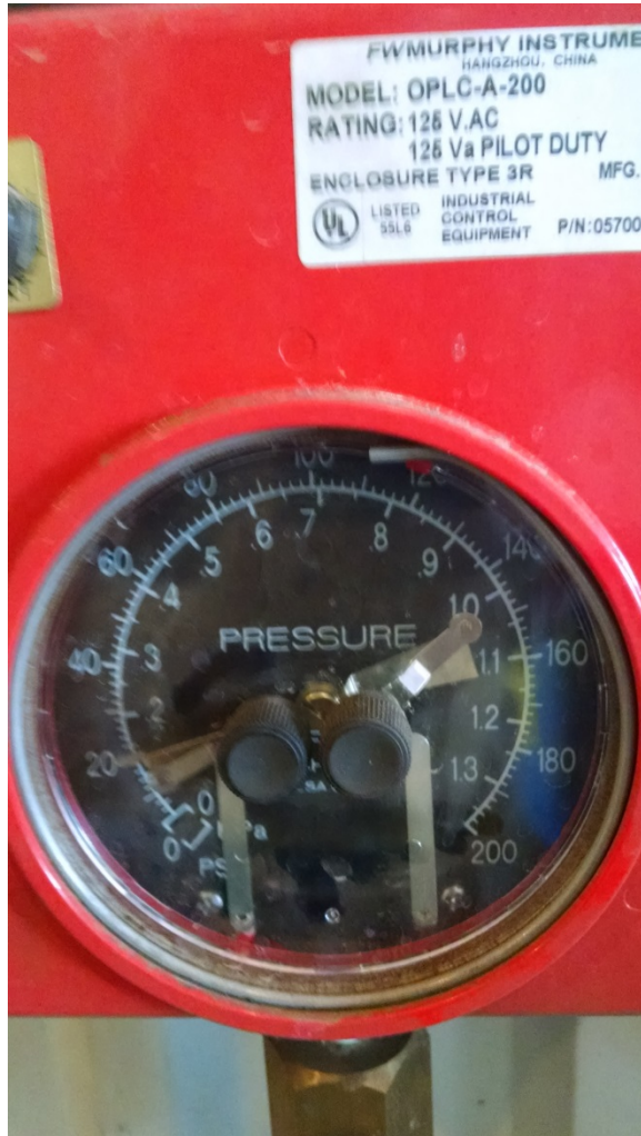
Low-pressure line gauge in Pump House
