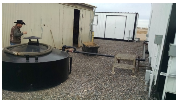
Above ground holding tank connected to pump house drainage and filter change units
