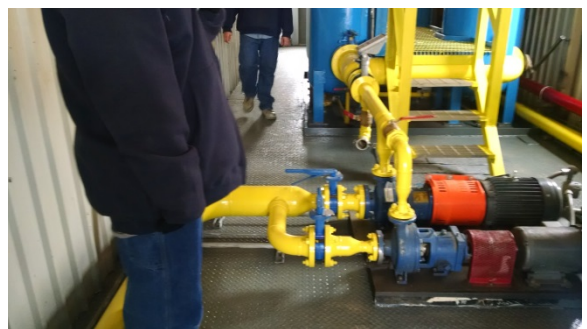
Yellow low-pressure & Red high-pressure lines in pump house
