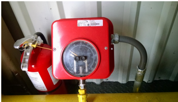
Low pressure gauge on Effluent Line w/ Fire Extinguisher
