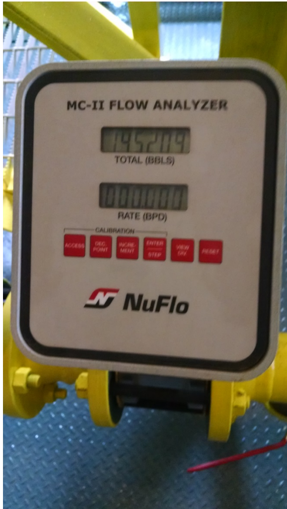
Flow Meter Totalizer in Pump House
