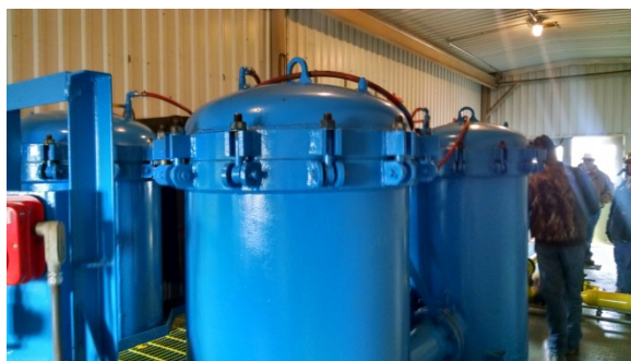
20micron/5micron Filtration Unit
