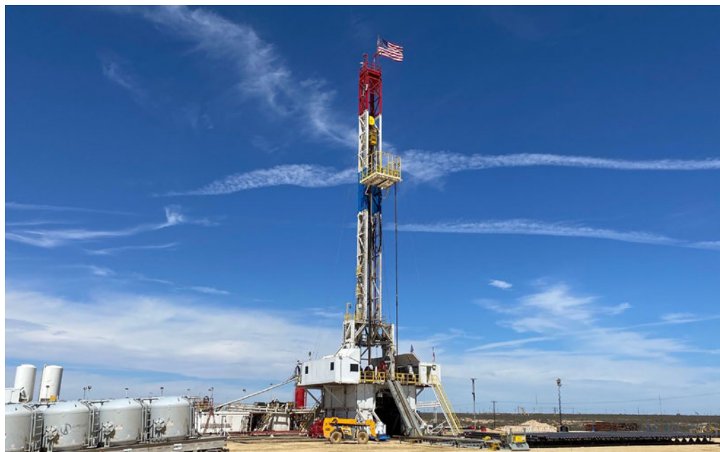
Images: Earthstone Drilling Rig Unit 410 Operating (2022)
