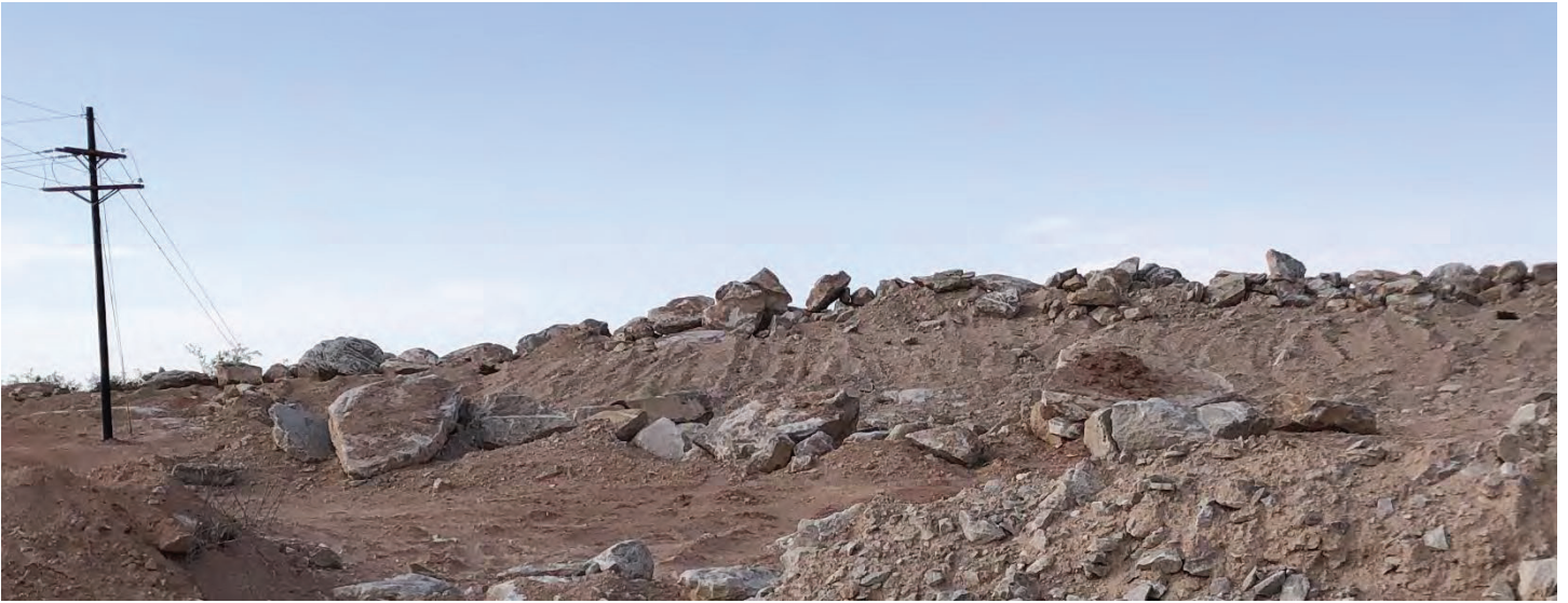
Figure 55A -The production pad due east of the containment area (see Figure 3A) lies on and in the Tamarisk Member of the Rustler Formation. During or just before 2019 the existing production pad (for a 1996 vertical well) expanded to allow for drilling one Devonian SWD and two horizontal wells. The pad expansion caused excavation of part of the massive, hard gypsum strata. Some blocks of gypsum on the side of the pad shown above are about the size of large pick-up trucks.
