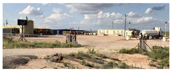
SP2- View northwest from RT 128 showing entrance to the recycling facility that serves the Mills Ranch in-ground Containment. The existing FED 128 containment is in the center of the image, below the powerlines. The avian protection netting makes the AST appear to have a cone-shaped top.
